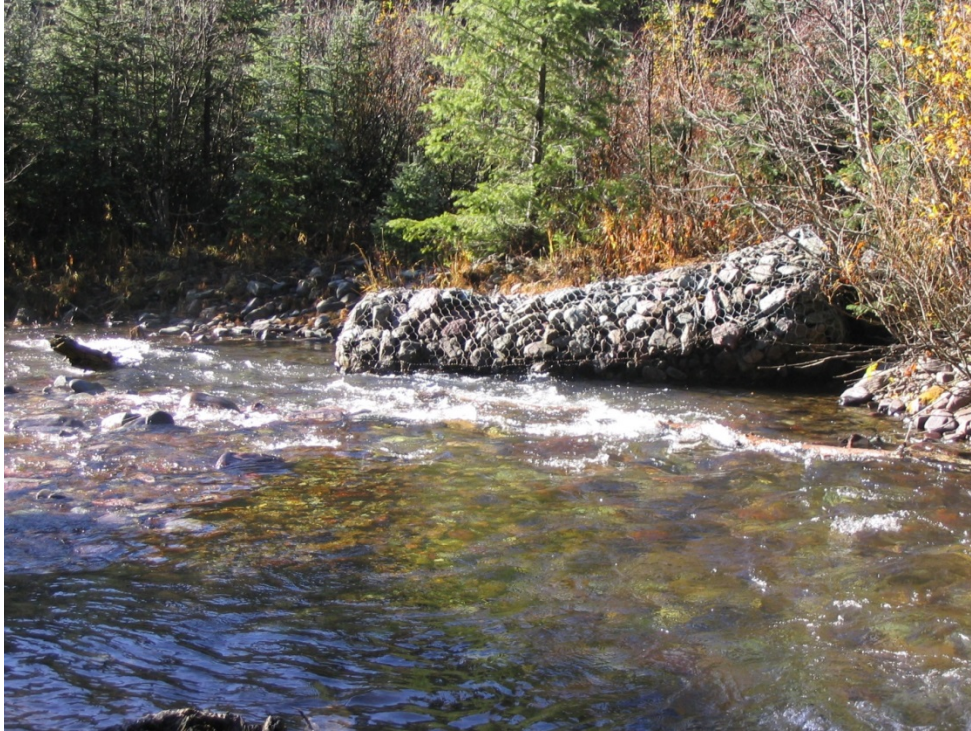
Photo 17: Main Stem Upper - Gabion for Fill Slope Protection
