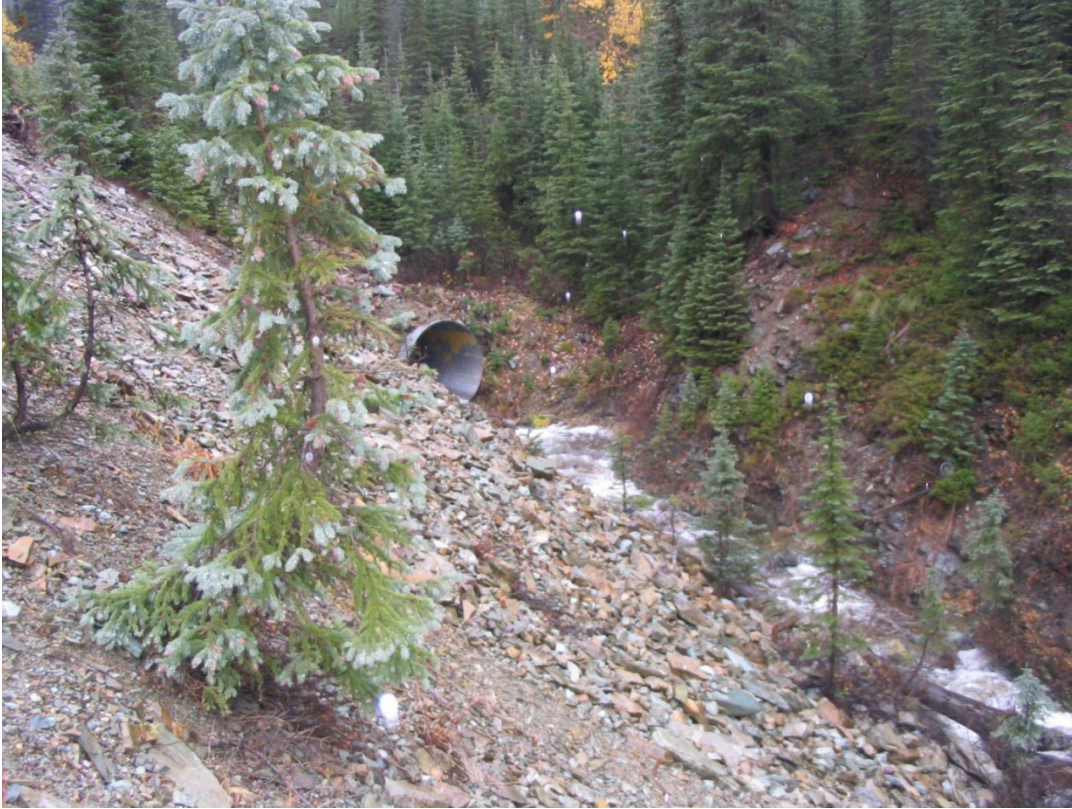
Photo 21: Fish Passage Barrier on Foundation Creek
