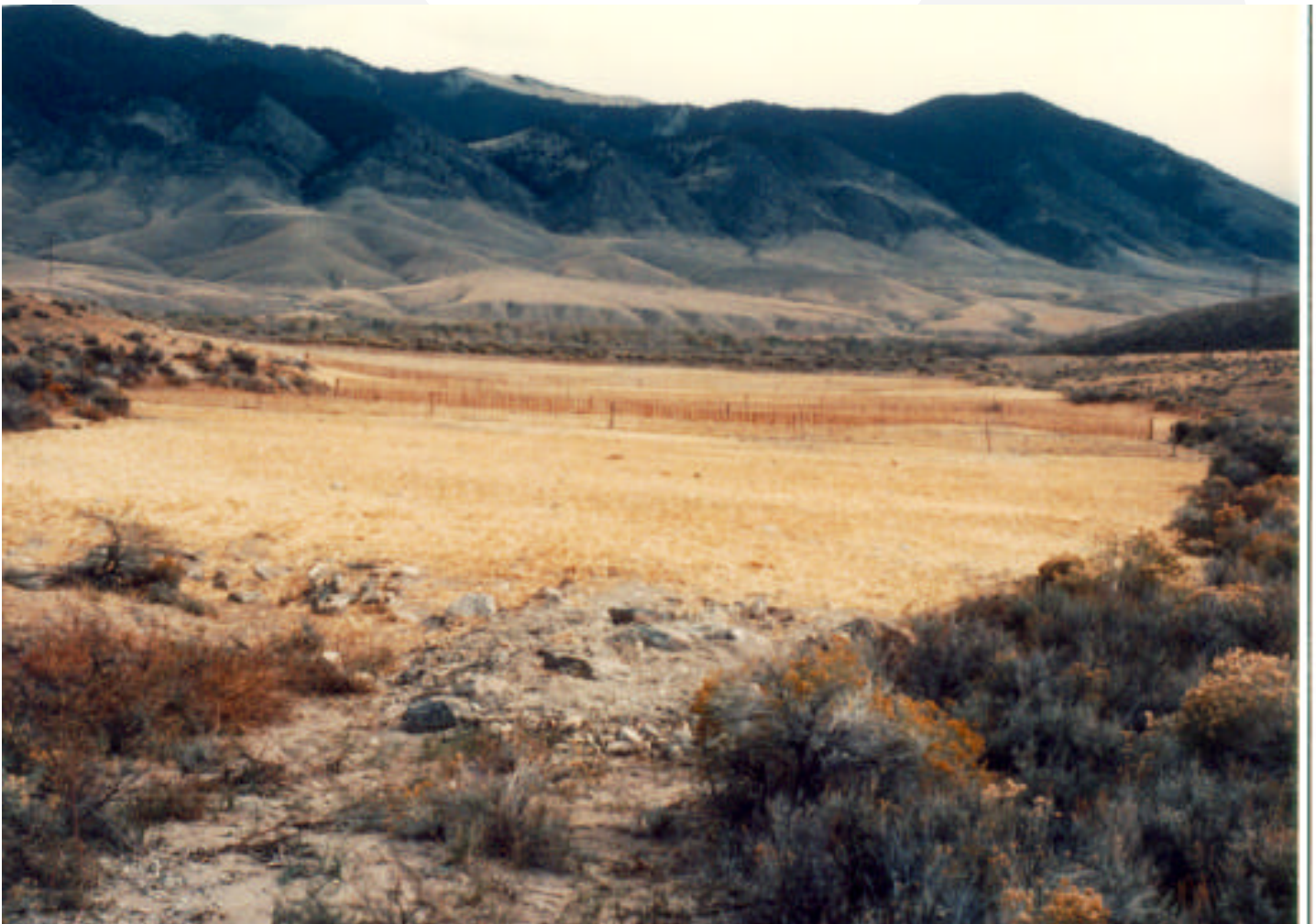
Glen Tungsten Mill site near Dillon, Montana just after reclamation. Straw mulch protects seed which will sprout in the next growing season.
