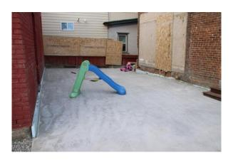
In April of 2018 an addition on a home in uptown Butte began to settle and pull away from the home. In July, after the removal of the addition, the ground failed leaving a 14 x 16-foot shaft almost 20 feet deep. The shaft connected to the abandoned Carrie mine which is located about 150 feet below the home. The AML Program stabilized the shaft, filled it with concrete and poured a separate concrete cap. The work took the remainder of 2018 and into 2019, saving the property.
