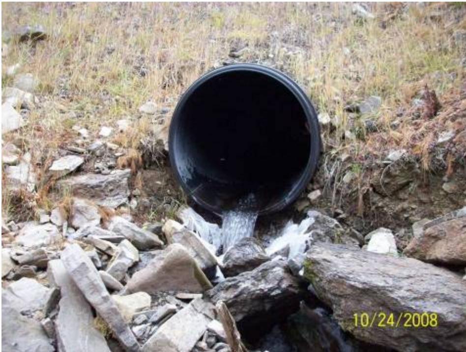
**Corrugated plastic culvert, fish passage barrier.**
