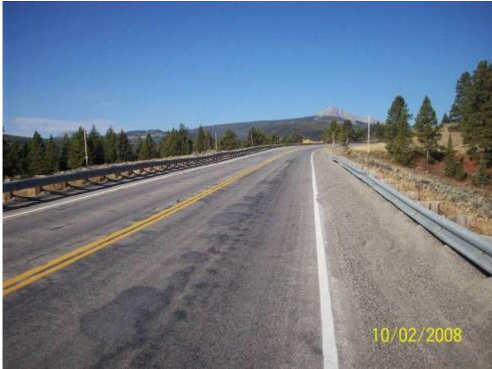
**Figure F-3. Typical build up of traction sand adjacent to a guardrail along Hwy 64. Crossing C12, North Fork West Fork Gallatin River.**
