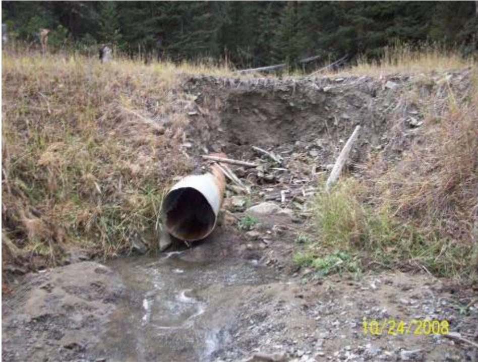
**Erosion of road fill material adjacent to perched corrugated steel culvert.**
