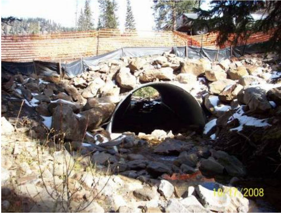
Photo 5. Silt fence installed at road crossing.
