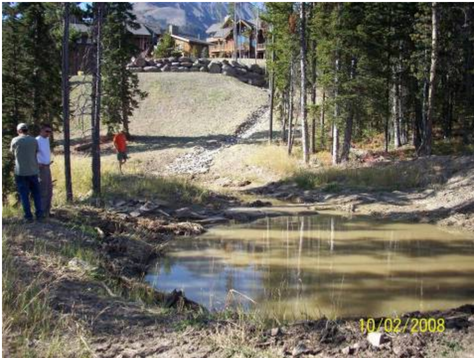
Photo 4. Rock lined storm water conveyance channel and sediment retention pond.
