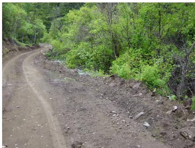
RAM#14. Off-cast material from grading piled directly above stream channel
