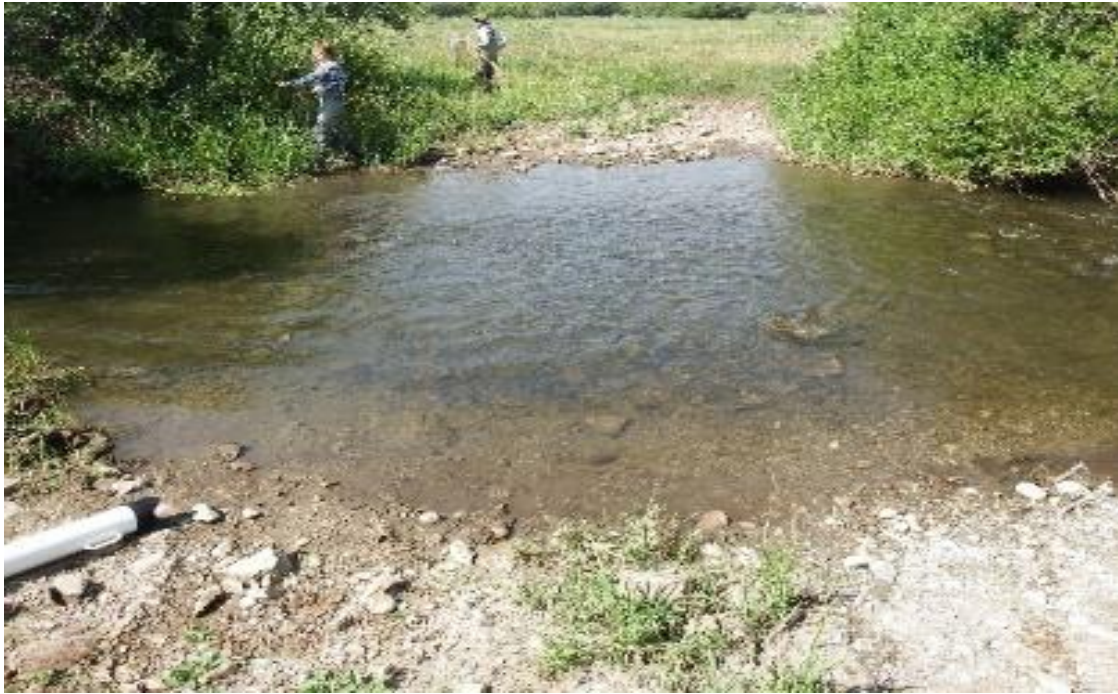
Figure 6-6. Unpaved crossing at site MDLG06-05a.
