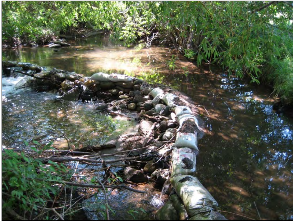
FIGURE 15. SANDBAGS DIVERTING WATER FOR WITHDRAWAL FOR RESIDENTIAL POND
