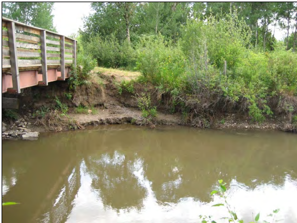
FIGURE 16. BANK EROSION DOWNSTREAM OF GALLATIN VALLEY LAND TRUST FOOTBRIDGE
