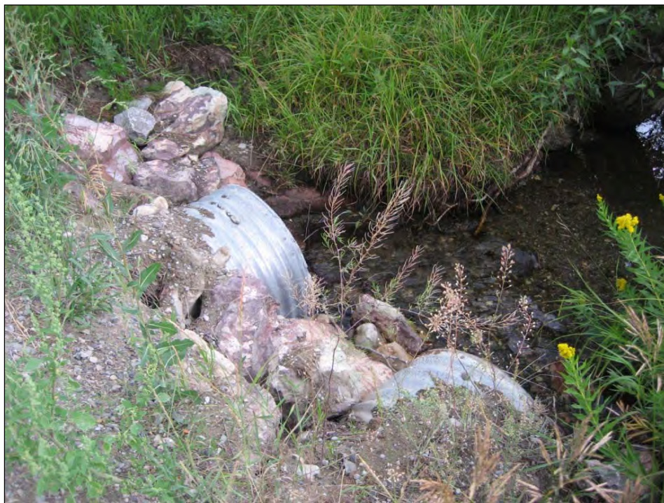
FIGURE 12. GRAVEL ON CULVERT AT GEE NORMAN RD
