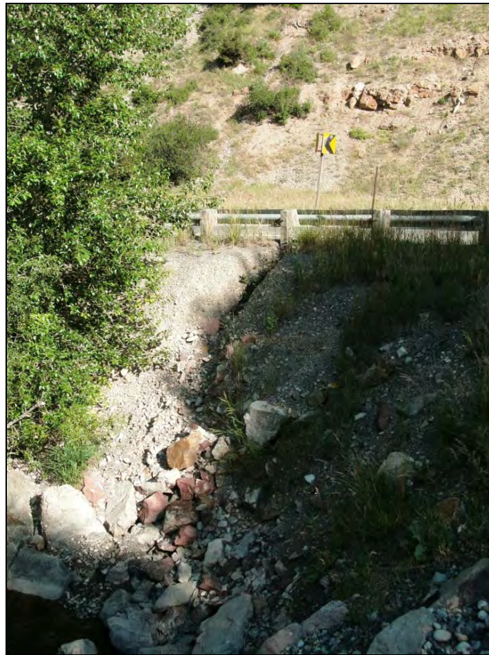
FIGURE 14. EROSION FROM POOR DRAINAGE OFF BRIDGER CANYON RD
