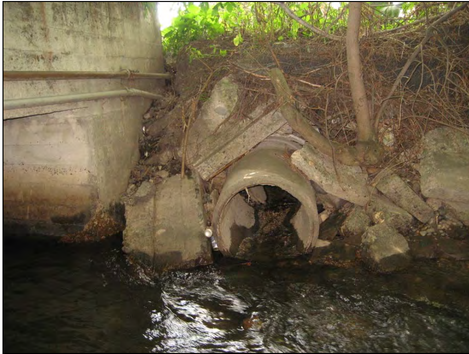
FIGURE 39. FLOWING STORMWATER PIPE DOWNSTREAM OF PEACH ST, WATER WARM AND SMELLED OF CHLORINE
