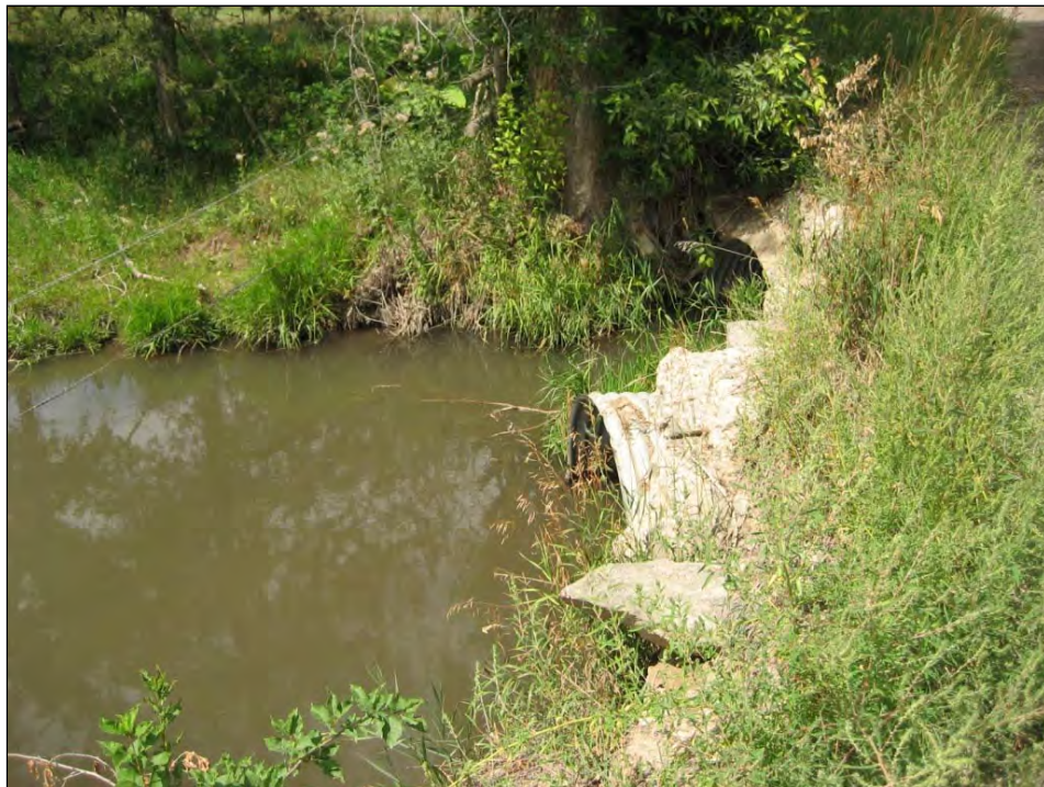
FIGURE 17. CULVERT DOWNSTREAM OF NORTH DRY CREEK ROAD; MINOR SEDIMENT SOURCE
