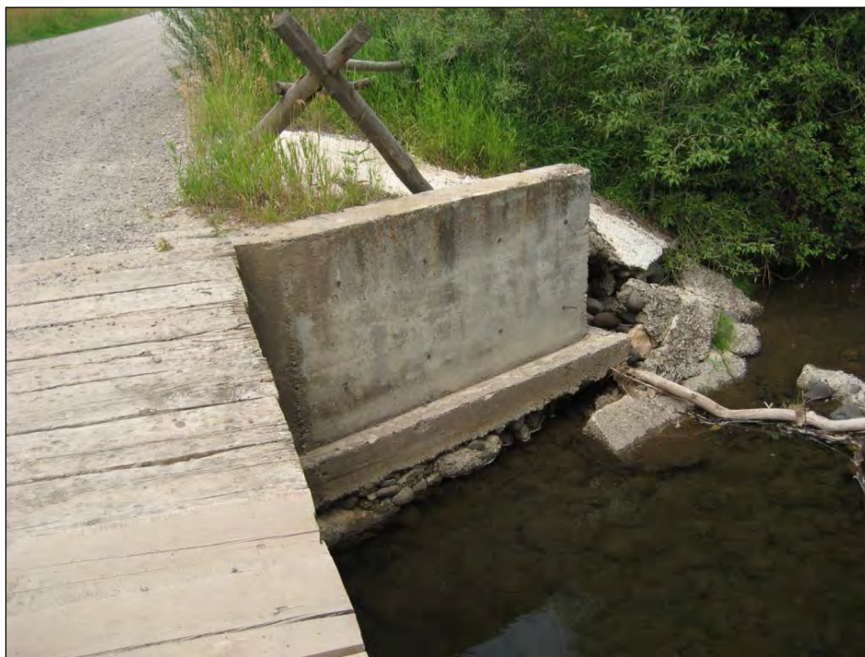
FIGURE 22. CONCRETE ABUTMENT AT ELK ROAD CROSSING
