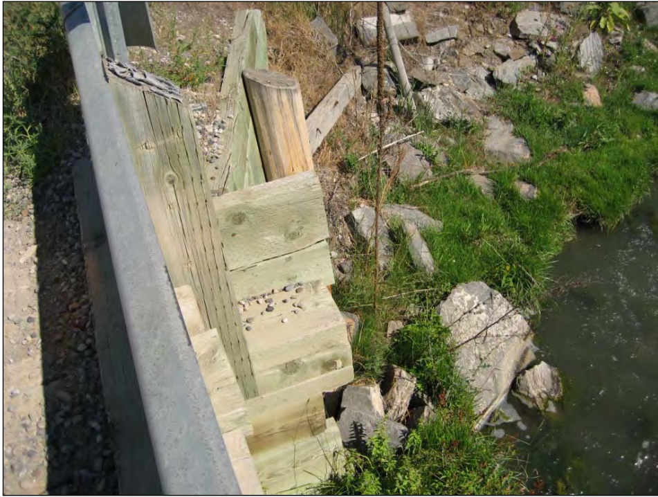
FIGURE 12. STABLE, WELL-VEGETATED ABUTMENT AT CANAL ROAD CROSSING
