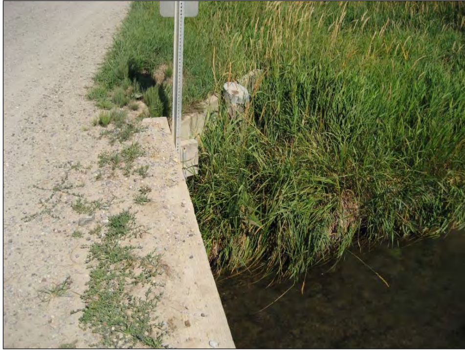
FIGURE 14. WELL-VEGETATED ABUTMENT WITH GRAVEL ON DECKING AT HAMILTON BRIDGE RD
