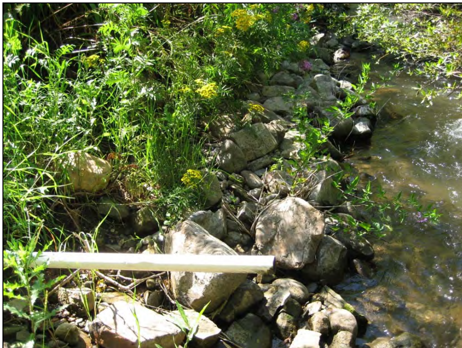
FIGURE 27. PVC PIPE ENTERING LEFT BANK JUST DOWNSTREAM OF SOUTH CHURCH ST. DRIPPING AT TIME OF ASSESSMENT
