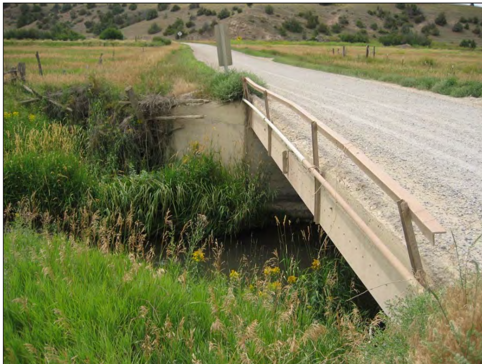
FIGURE 13. GRAVEL ON BRIDGE DECKING AT NORTH DRY CREEK ROAD WITH STABLE, WELL-VEGETATED ABUTMENTS
