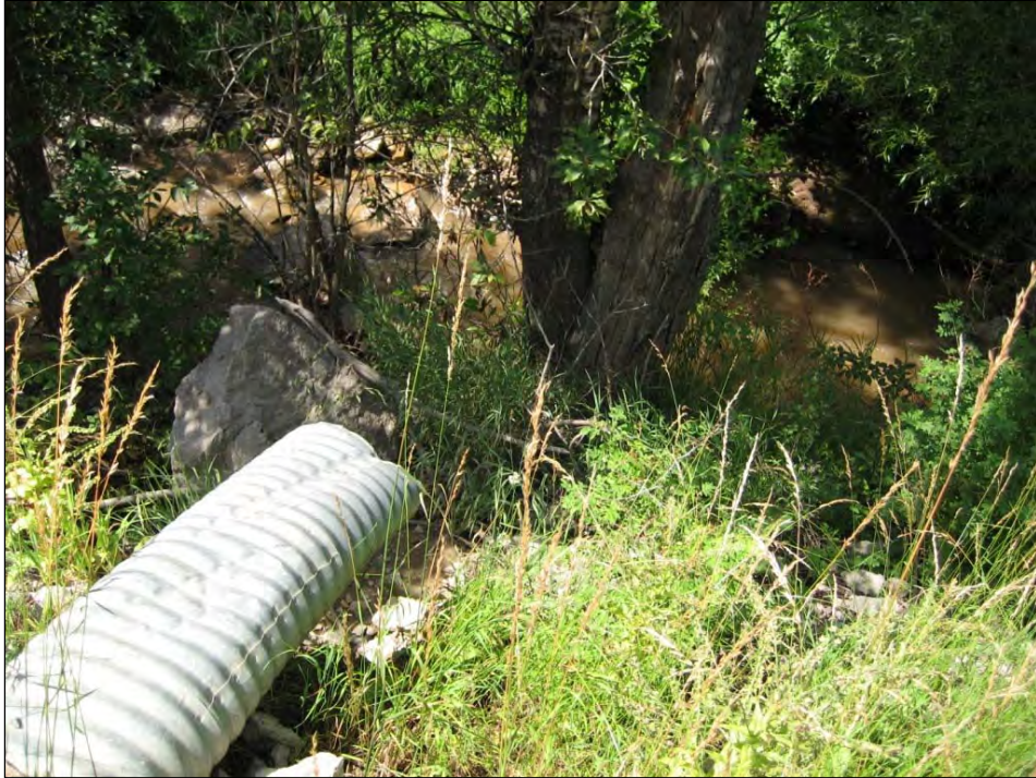
FIGURE 17. PIPE DRAINING BEAR CANYON ROAD DITCH WITHIN REACH BEAR 03 N
