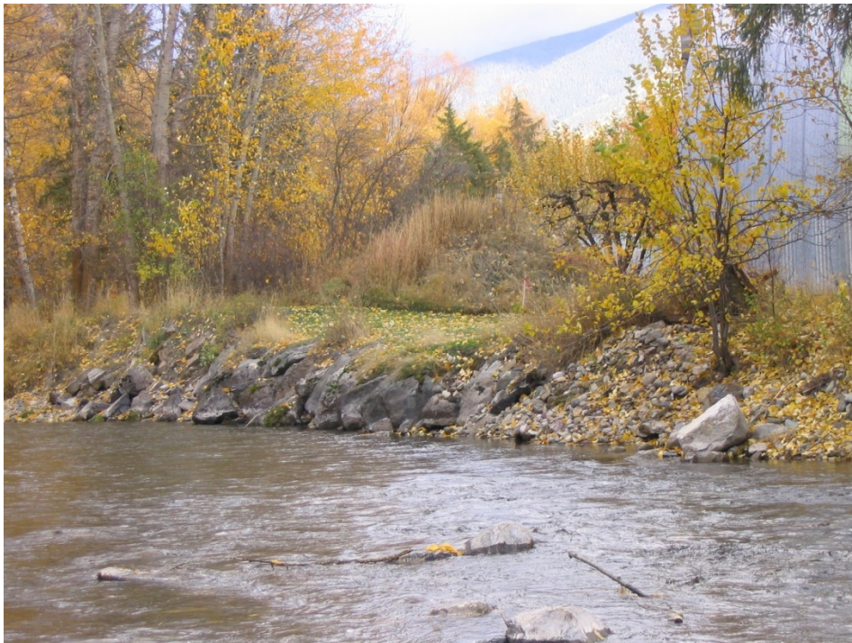
Photo 20: Main Stem Lower - Bank Armoring
