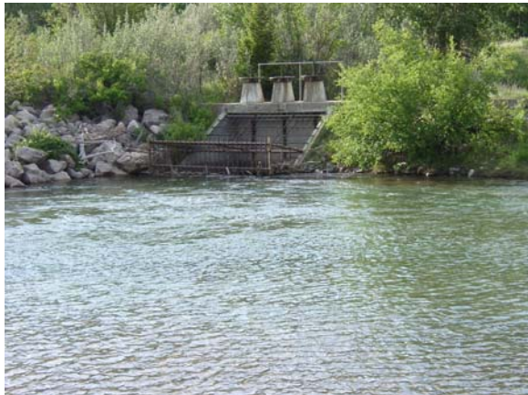
Figure 2-5. Flat Creek diversion gate structure (view from Dearborn River)
