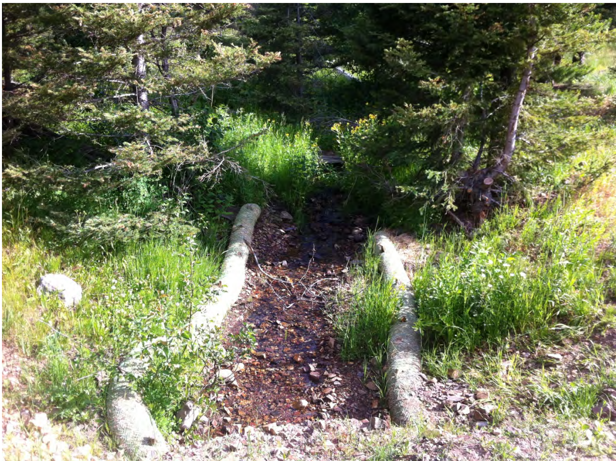
Figure 5-1. Culvert replaced by the US Forest Service in 2012
