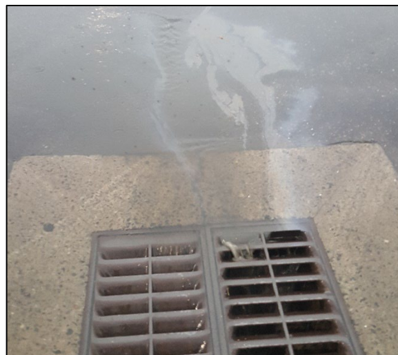
Figure 3-10: Impervious surfaces such as asphalt prevent rain and snow from infiltrating through soils and into groundwater. Instead, precipitation runs off over the land, picking up pollutants along the way. Storm drains offer some level of treatment before discharging the runoff as surface water.
