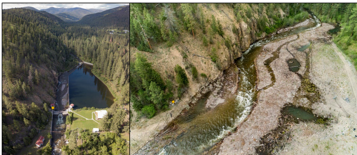
Figure 3-4: Before (left) and after (right) the Rattlesnake Creek dam was removed to restore hydrologic regime and fish passage. Photo credit: project partners - City of Missoula and Trout Unlimited.
