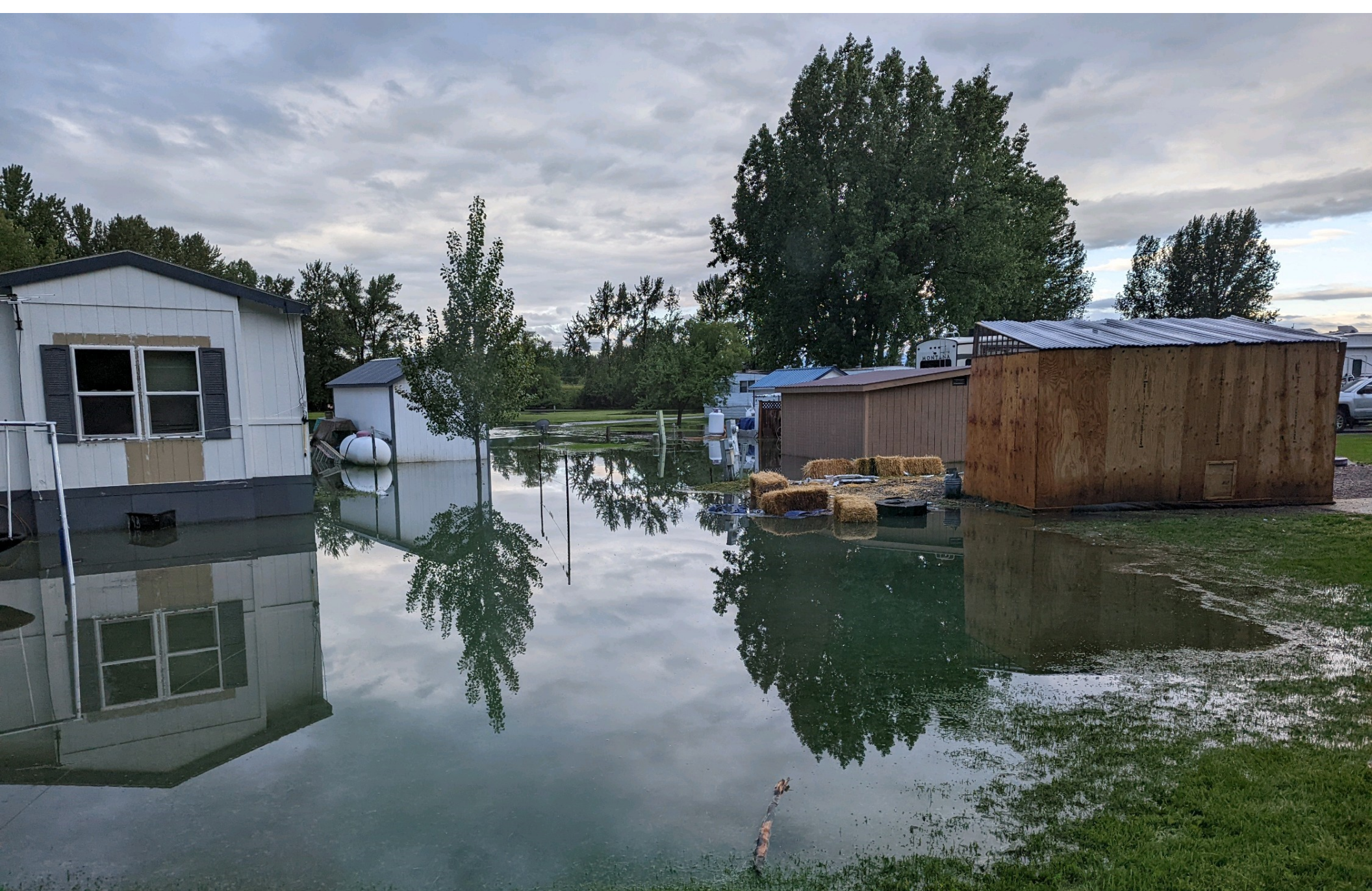
These photos are from the Cynthia Lane area in 2022. Flooding exacerbates the septic system contamination issues and well as public health risks.
