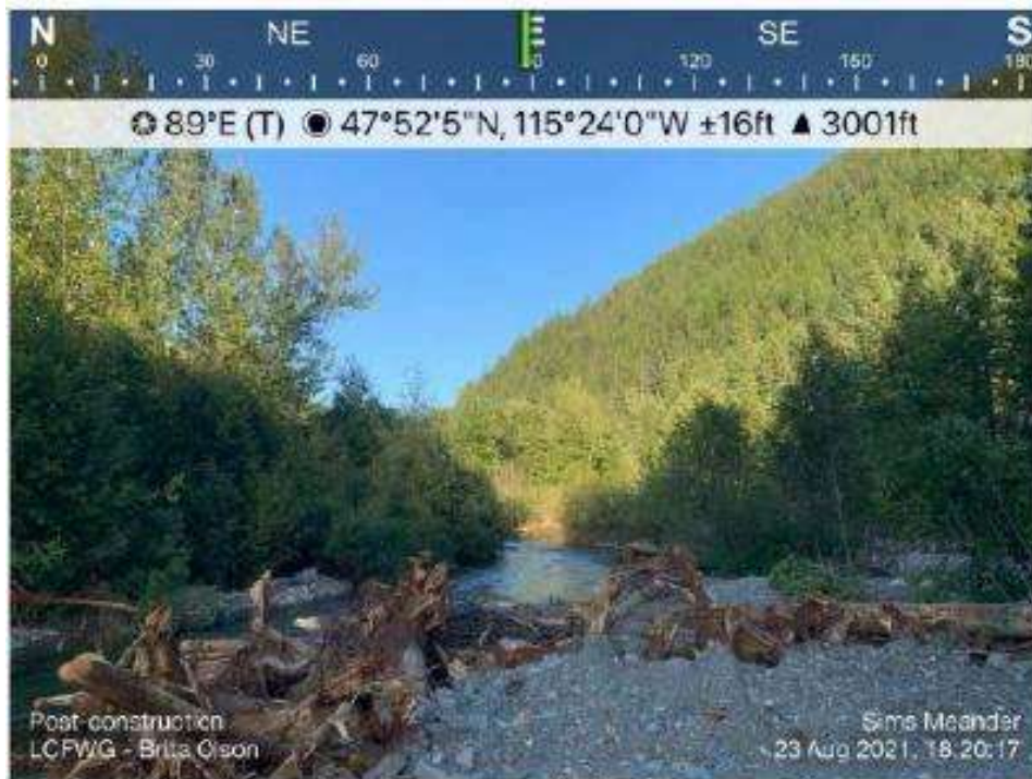
Large woody debris was placed in the stream channel to help the river disperse onto its floodplain during high flows, and to create varied in-stream habitat. (Pre- [top] and Post-Construction Photos: Lower Clark Fork Watershed Group)
