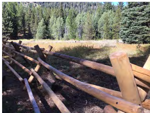
Jack leg fencing installed to restrict the expansion of a campground into a sensitive
