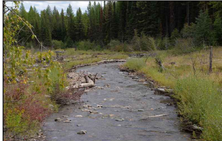
TYPICAL CONSTRUCTED STREAMBED THROUGH A RIFFLE FEATURE
