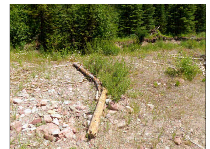
EXAMPLE OF A CONSTRUCTED VEGETATED BRUSH TRENCH
