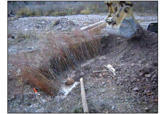
EXAMPLE OF A VEGETATED BRUSH TRENCH INSTALLATION
