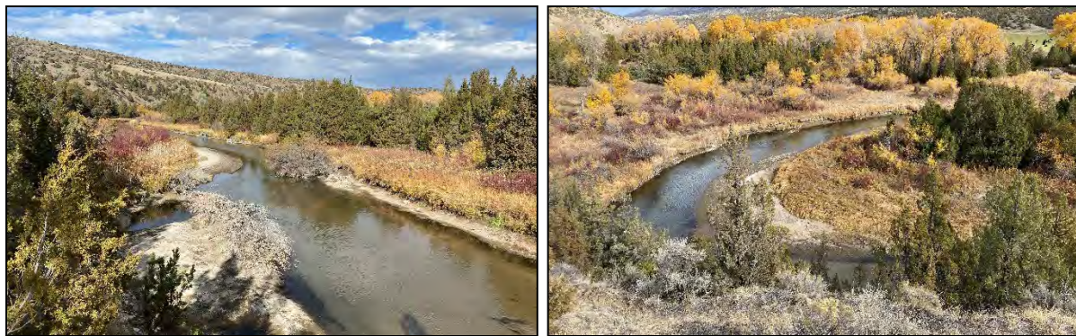
Figure 2-11. Sediment deposition and bar formation upstream of Shaw Diversion Dam (left). Active bank erosion along outside meander bend (right).
