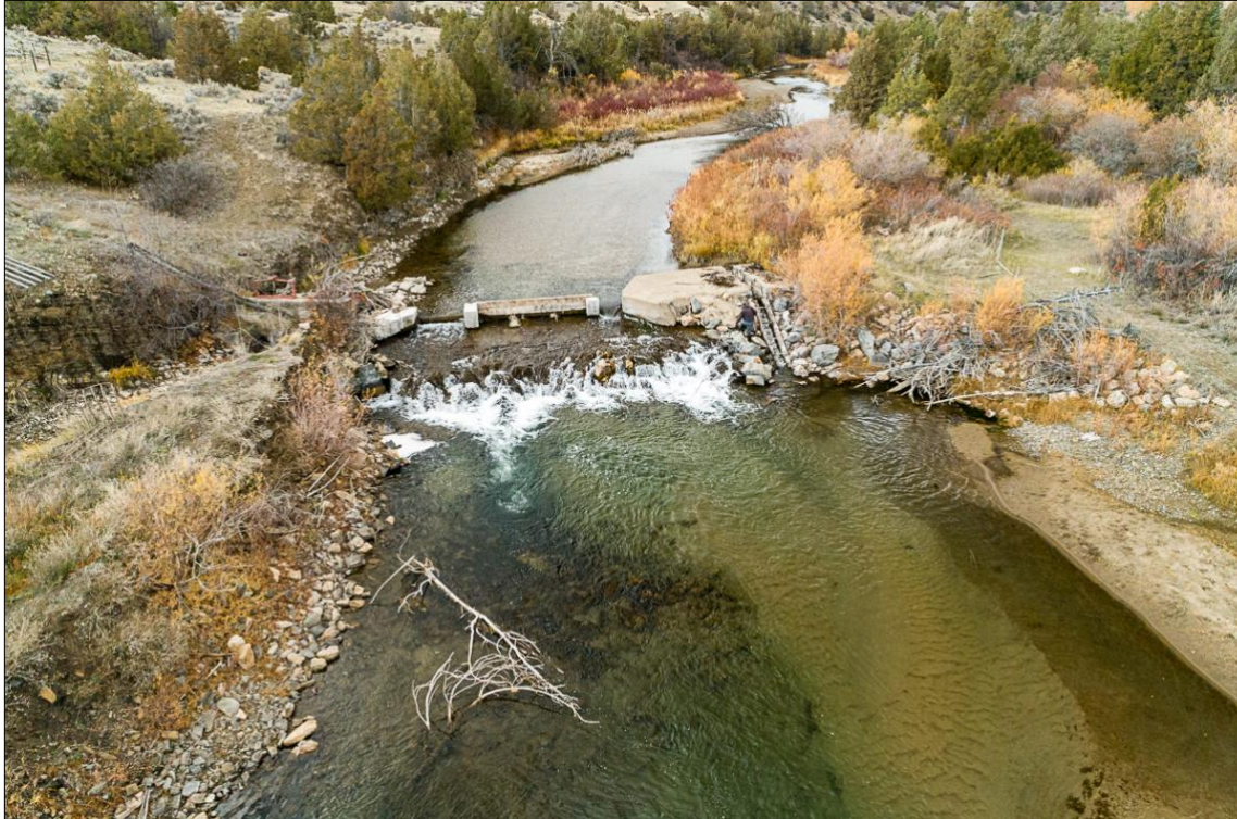
Figure 1. The Shaw Dam has disrupted natural processes, such as sediment transport and deposition, for over a century. Restoring these processes and reconnecting the floodplain to improve non-point source (NPS) pollution are key goals of the project.
