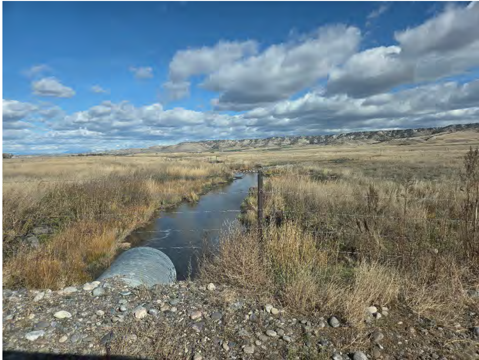
Figure 9: One of several irrigation ditches that convey water diverted from the Madison River. Even outside of irrigation season they function as “stream ditches”, flowing year-round due to groundwater inputs.
