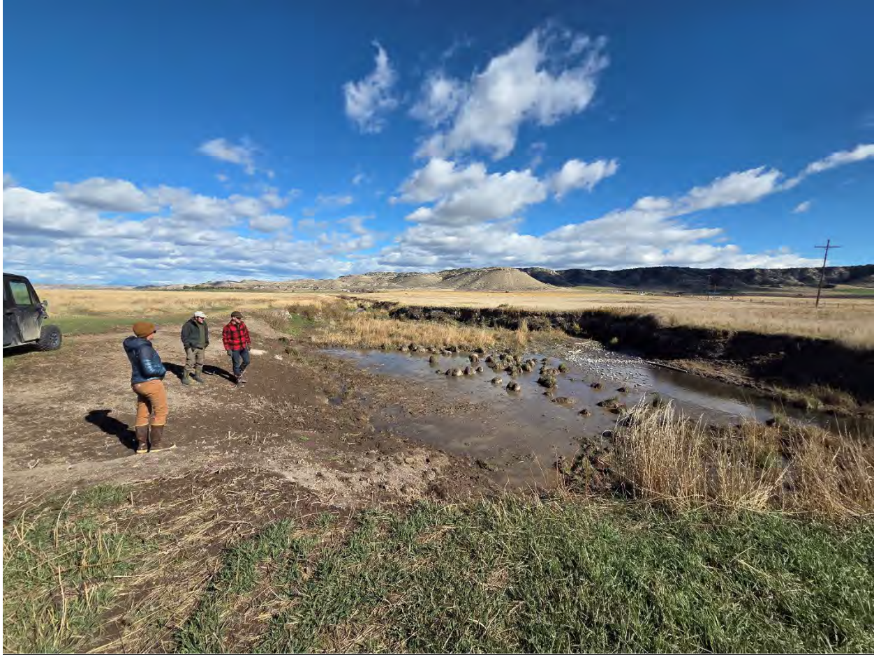
Figure 1: Eroding stream banks caused by historic overgrazing along Spring Creek, a tributary to Rey Creek.
