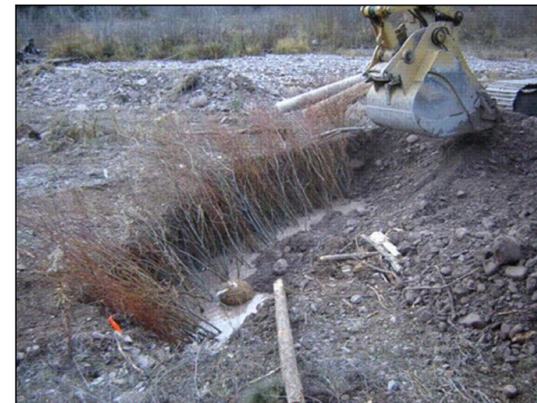
EXAMPLE OF A WILLOW TRENCH INSTALLATION
