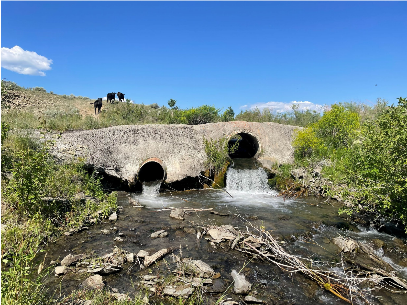
Figure 2. Culvert outlets.
