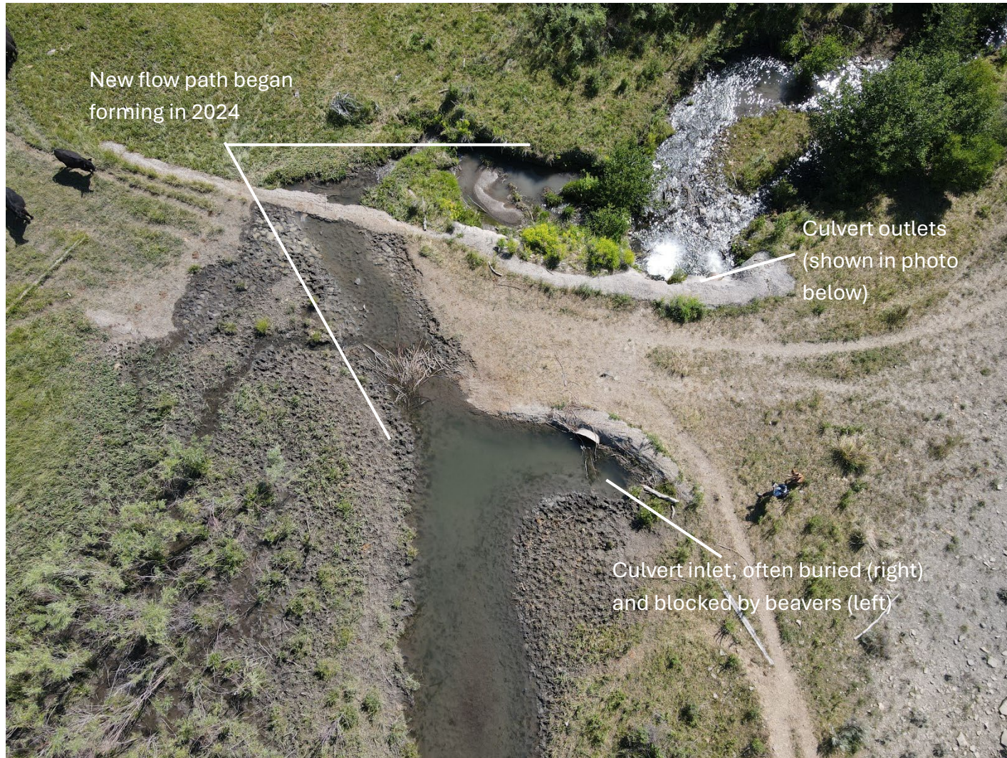
Figure 1. Drone photo of the concrete structure to be removed.
