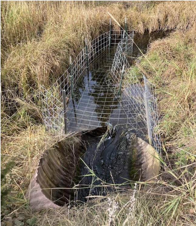
Figure 8. Exclusion fence to prevent culvert plugging on a Lolo National Forest Access Road, Seeley Lake, within the Clearwater WRP.
