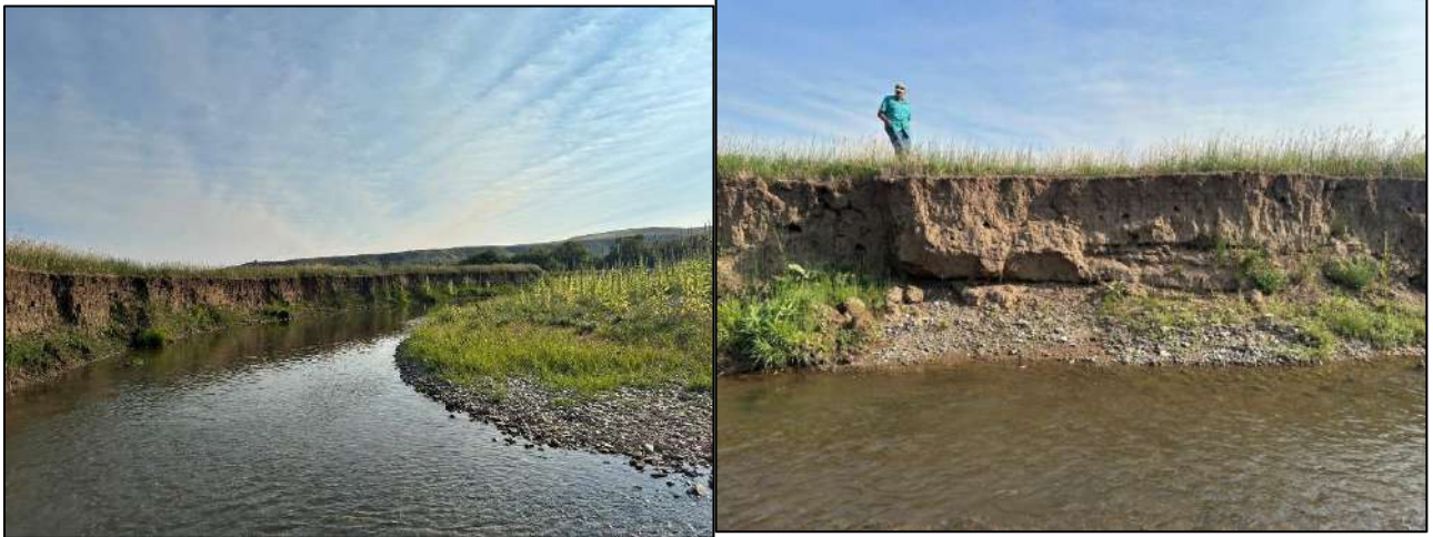
Figure 20. Eroding streambank in Phase 1 project area.
