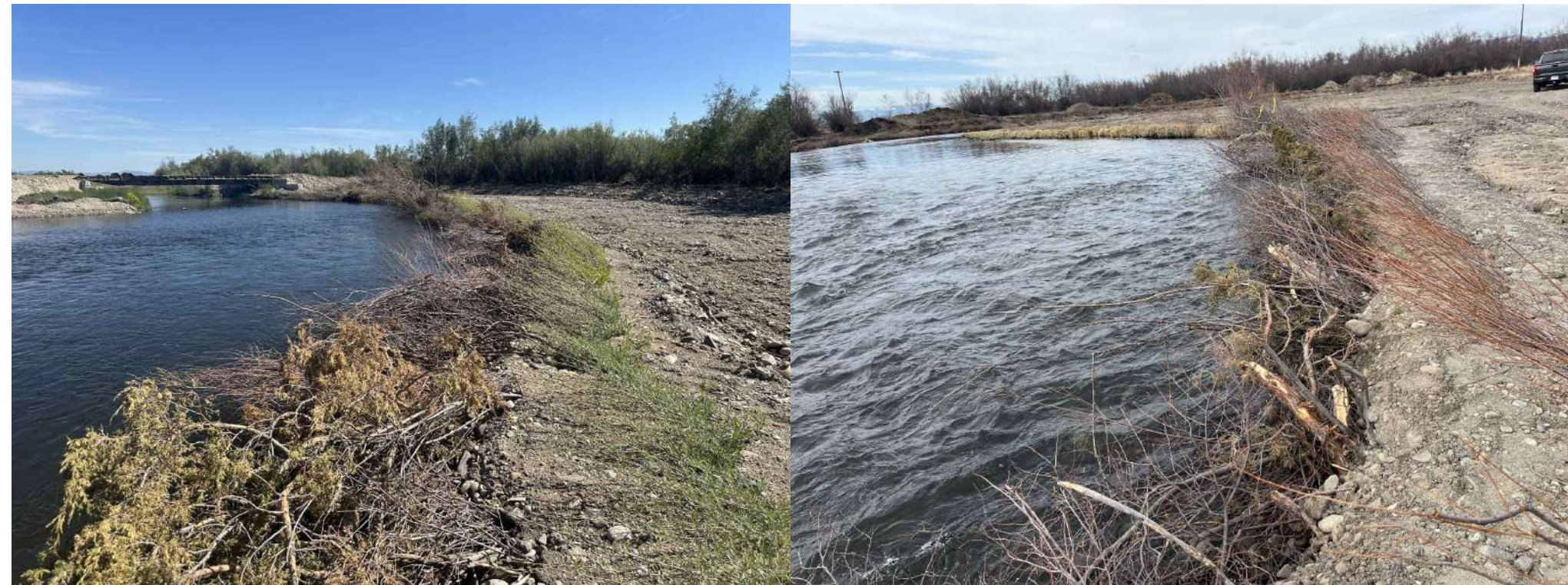
BRUSH MATRIX STREAMBANK TREATMENT EXAMPLE PHOTOS
