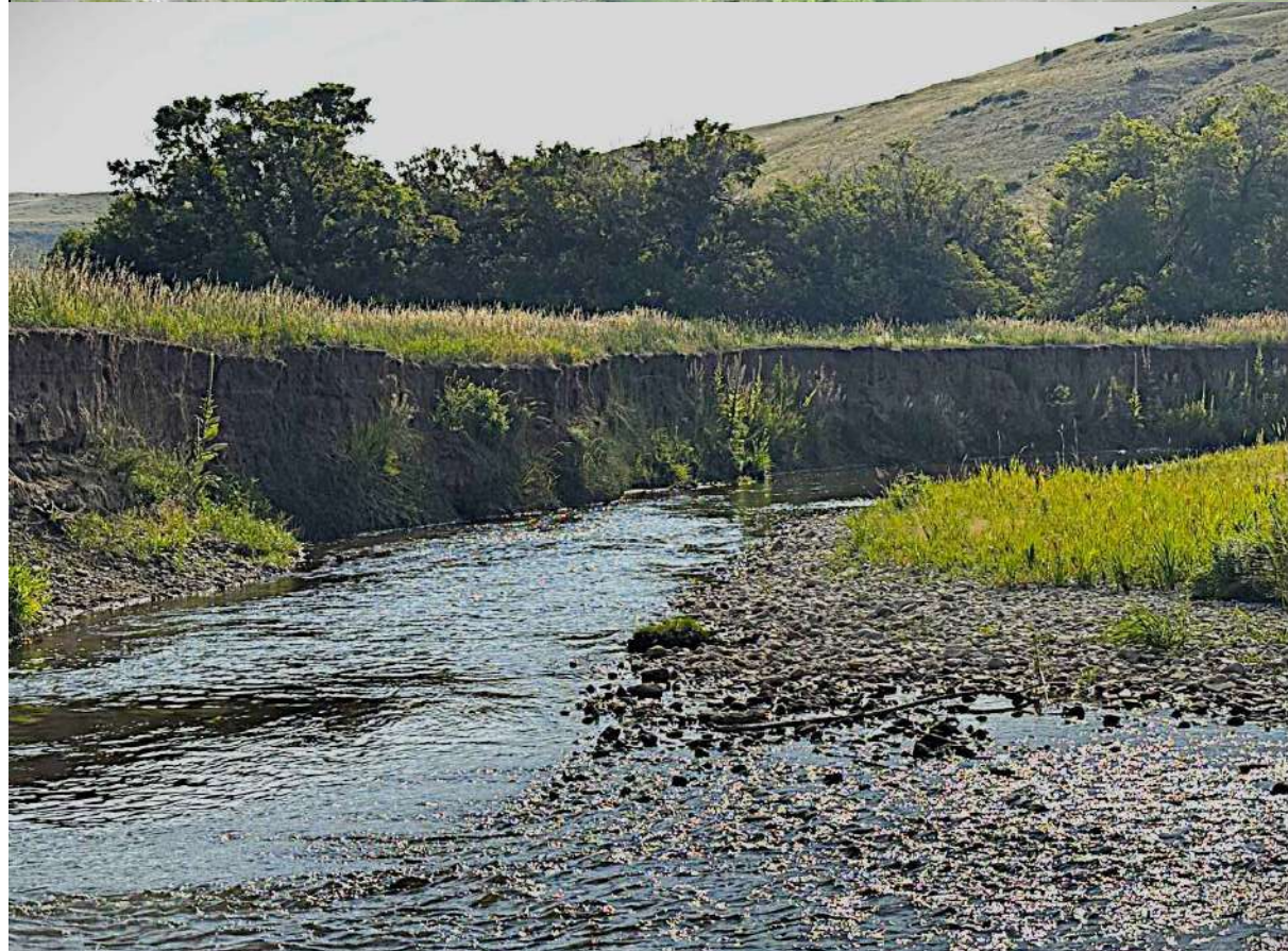
HIGH LATERAL ERODING BANK EXAMPLE PHOTO PHOTO TAKEN ON 8/22/2025 SHOWING THE LATERALLY ERODING BANK IN HOUND CREEK PHASE 1 PROJECT AREA. THIS BANK WOULD BE LAYED BACK AND THE EXISTING CHANNEL SEGMENT WOULD BE ABANDONED AND FILLED TO CREATE CONNECTED FLOODPLAIN.
