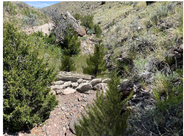
Figure 5: Here is another artist's rendering of what this area will look like in 4 to 6 years. Again notice the Sediment Capture Structure made of Rocks and woody debris
