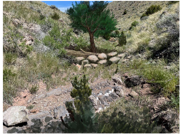
Figure 3: Here is an artist's rendition of what this site will look like in Ten Years. Notice the rock and wood Sediment Catchment Structure
