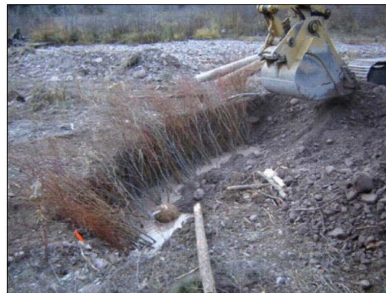
EXAMPLE OF A VEGETATED BRUSH TRENCH INSTALLATION
