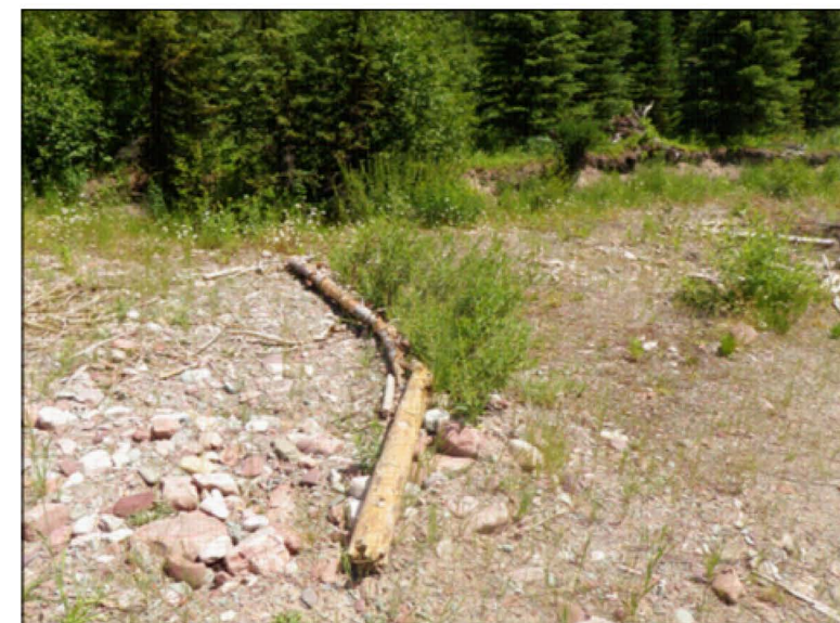
EXAMPLE OF A CONSTRUCTED VEGETATED BRUSH TRENCH
