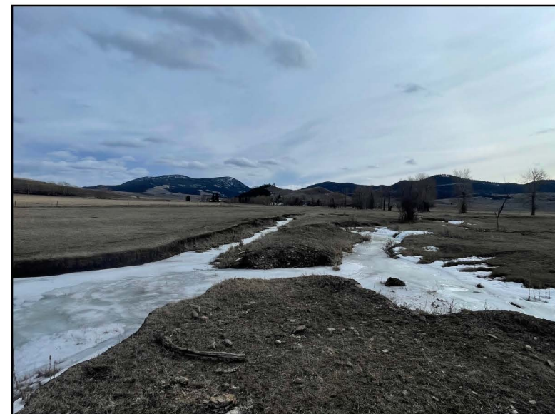
VIEW OF EXISTING STRAIGHTENED CHANNEL (PHOTO LEFT) AND HISTORICAL CHANNEL ALIGNMENT (PHOTO RIGHT) IN REACH 2 . THE EXISTING BERM HAS BREACHED RESULTING IN A BIFURCATED CHANNEL AND SEASONAL DEWATERING.
