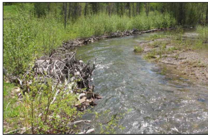
TYPICAL CONSTRUCTED STREAMBED THROUGH A RIFFLE FEATURE
