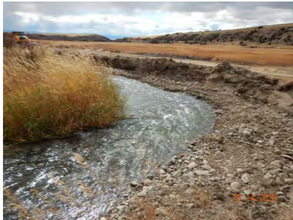
STEP 1 - TYPICAL GRAVEL BASE LAYER
