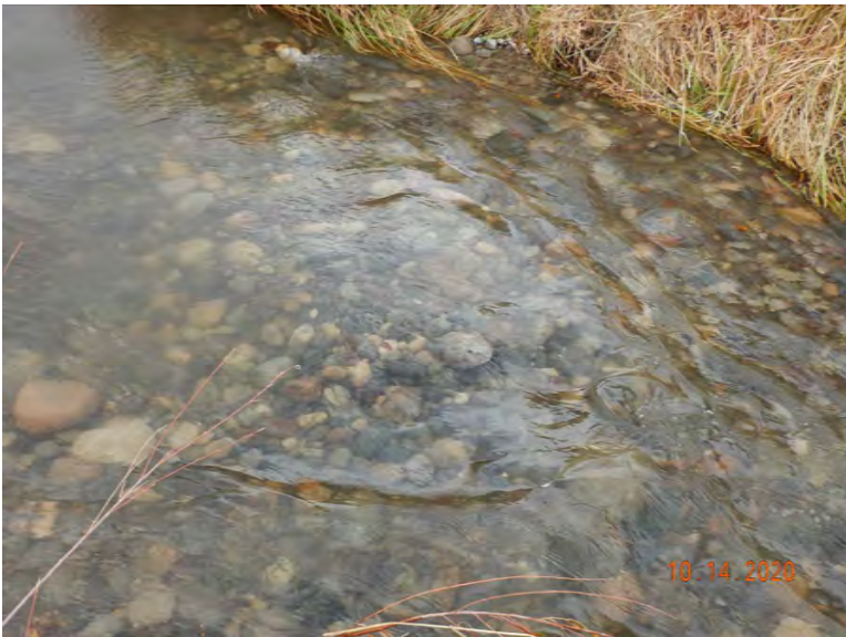
RIFFLE AGGRADATION
