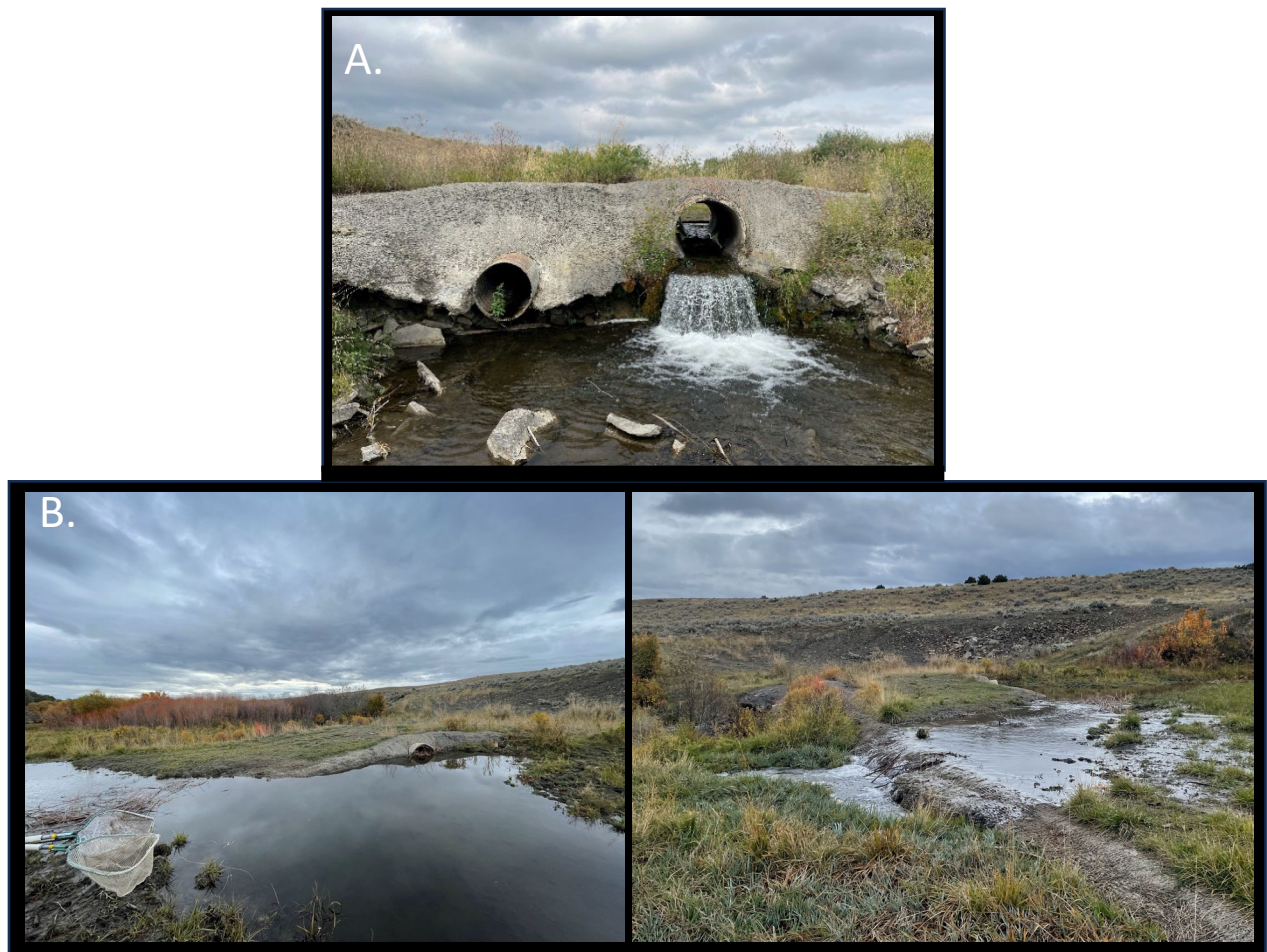
Figure 2. A) Looking upstream at the dam in 2022 before beavers blocked the second culvert. Erosion underneath the cement structure is evident. B) In 2023 beavers blocked the culvert and the stream began forming a new channel to the north of the existing channel and culvert.
