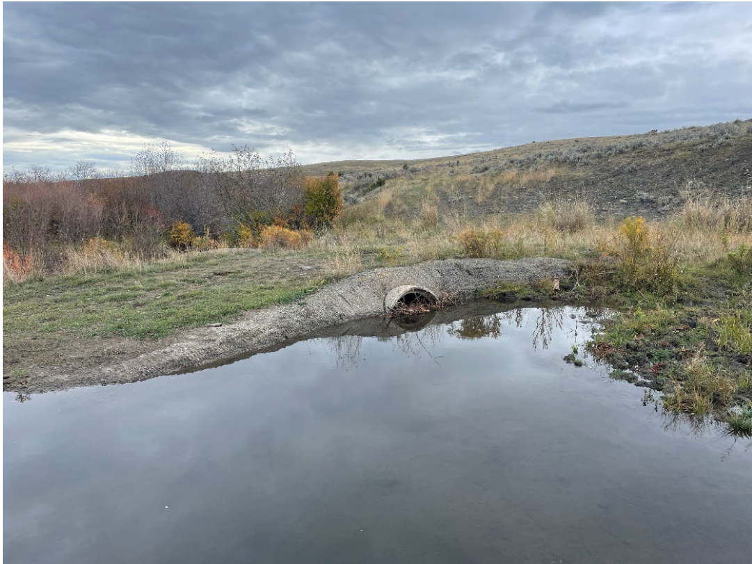
Looking downstream at the dam with the culvert blocked by beaver activity.
