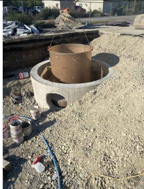
Installing Treatment Unit
