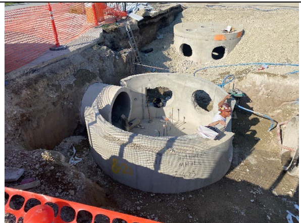
Installing Treatment Unit
