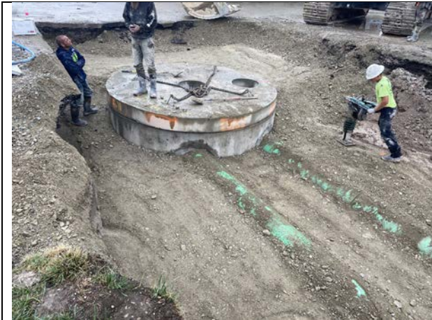
Backfill and compaction around the connection piping and treatment unit
