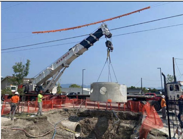
Installing Treatment Unit
