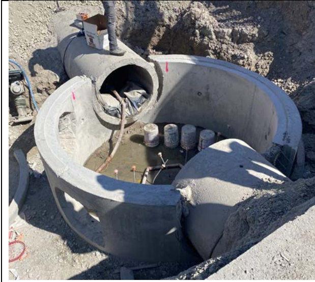
New Storm Main Pipe Connection to Existing Storm Pipe
