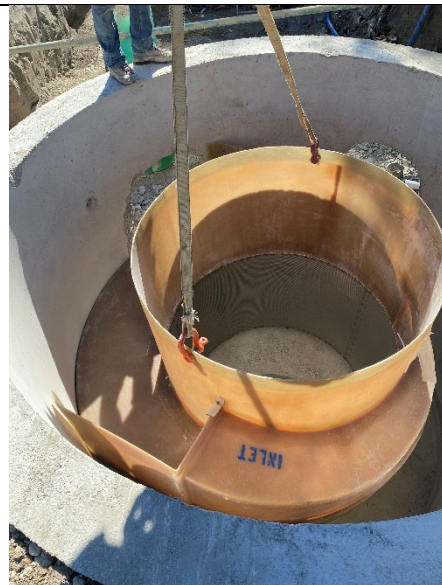
Installation of Treatment Unit internals
