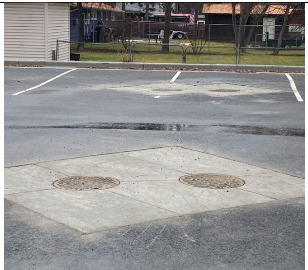
Completed construction – Near manholes are the Treatment unit, Far manholes are the diversion structure
