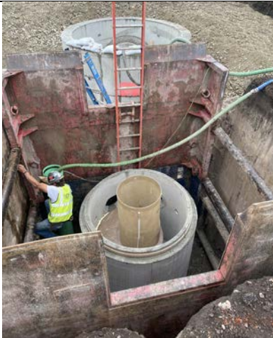
Installing Treatment Unit
