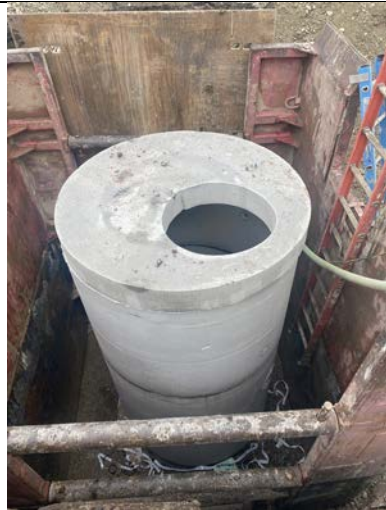
Installing Treatment Unit
