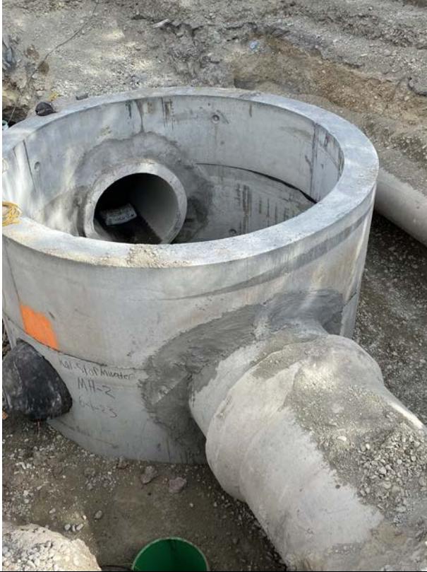
Manhole connection to existing Storm Main Pipe
