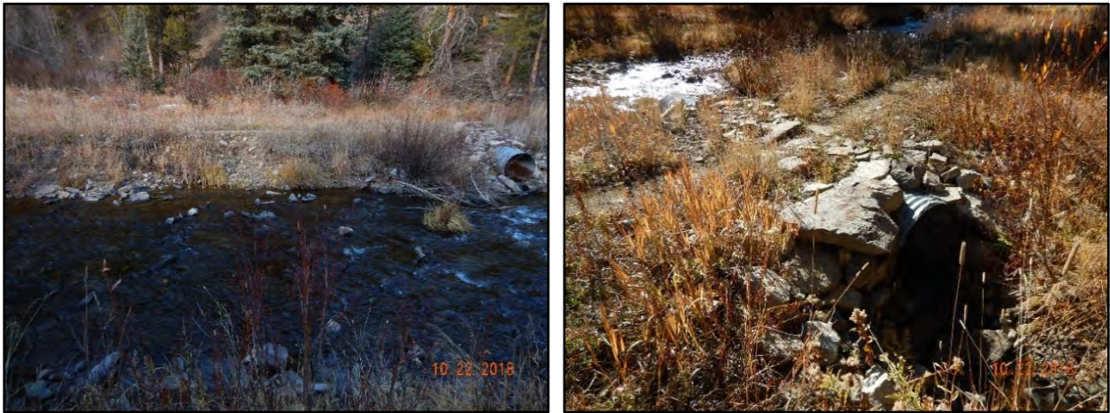
Figure 14. Streambank Erosion and Culvert along Former Logging Road and Current Trail
