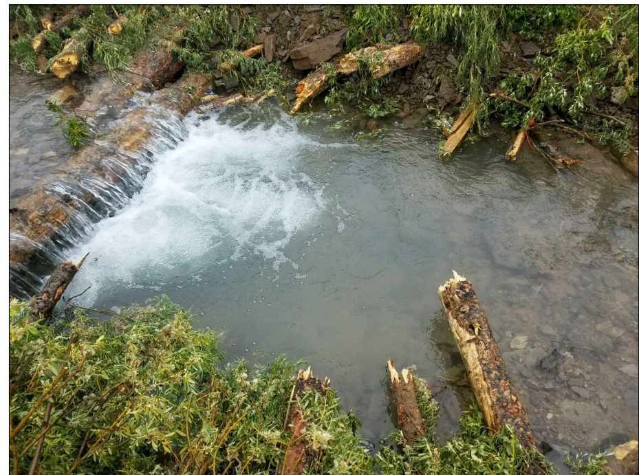
EXAMPLE OF A CONSTRUCTED LOG STEP POOL
