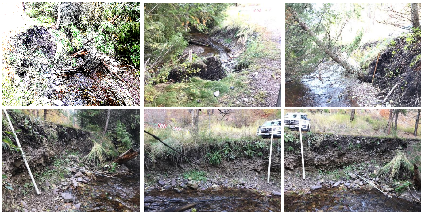
Figure A.18: Reach 8 – significant bank erosion section along streamside Forest Road. No. 123.
