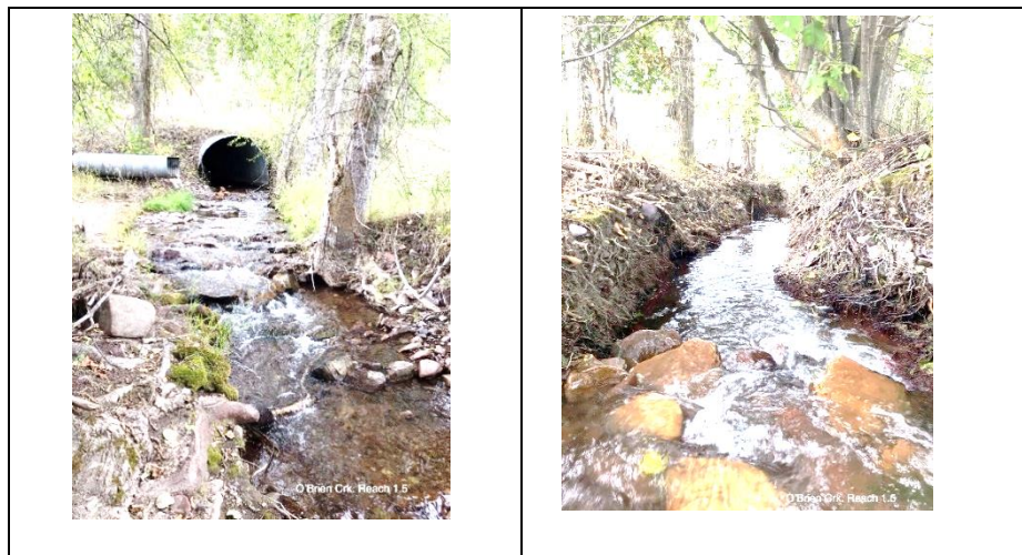
Figure A.10. Road crossing to O'Brien Creek Meadow Subdivision and critically undersized and actively downcutting segment downstream of the subdivision crossing and upstream of Blue Mtn. Rd.
