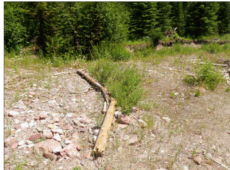
EXAMPLE OF A CONSTRUCTED VEGETATED BRUSH TRENCH
