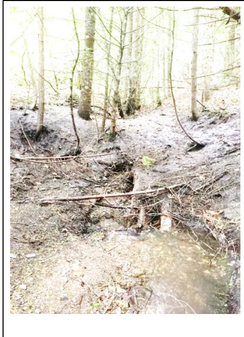
Figure A.22: Failed log culvert on jammer road in Upper O'Brien Creek jammer road system.
