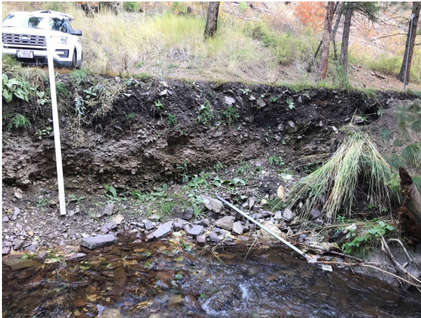
The road failure is 6 feet in height and 54 feet long.
