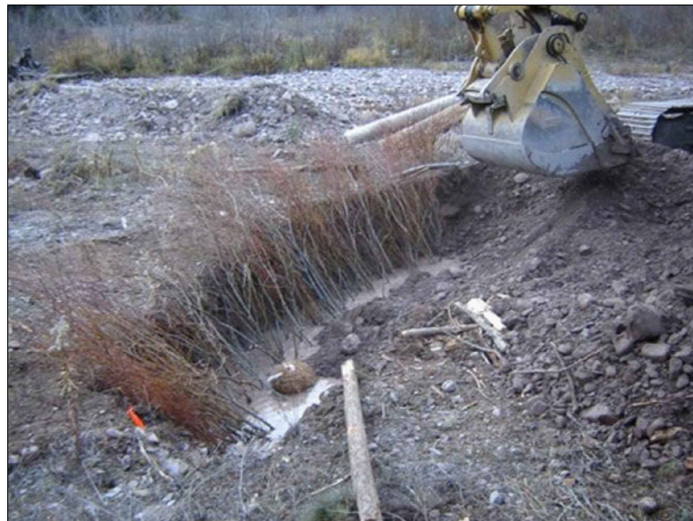
EXAMPLE OF A VEGETATED BRUSH TRENCH INSTALLATION
