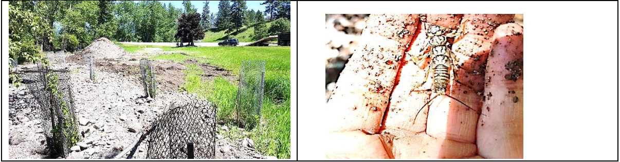
Figure A.23. Reach 3 - 2019 Emergency Channel Remediation conducted by O'Brien Creek HOA with tree donation from Hillsdale Estates. Mass failure and temporary remediation with large tree toe protection; salvage of large rainbow trout and macroinvertebrates.
