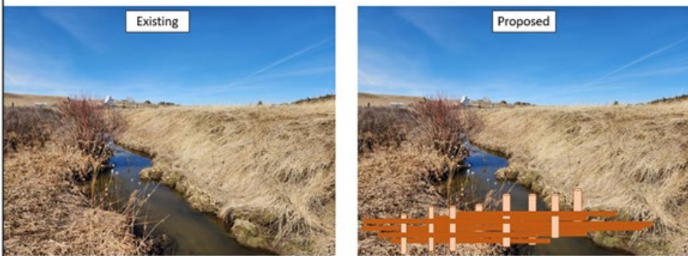
Figure 9: A photo of Camp Creek with depictions of a Beaver Dam Analog.
