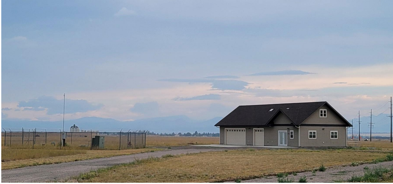
Figure 4: Well and Pumping Facilities Building
