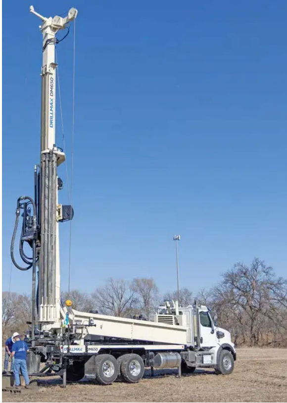
Figure 1: Image of Drill Rig
