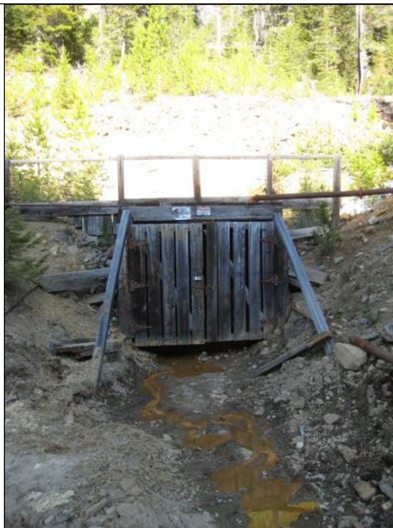
Figure 5-3b. Galena Creek Mine Drain/Adit
