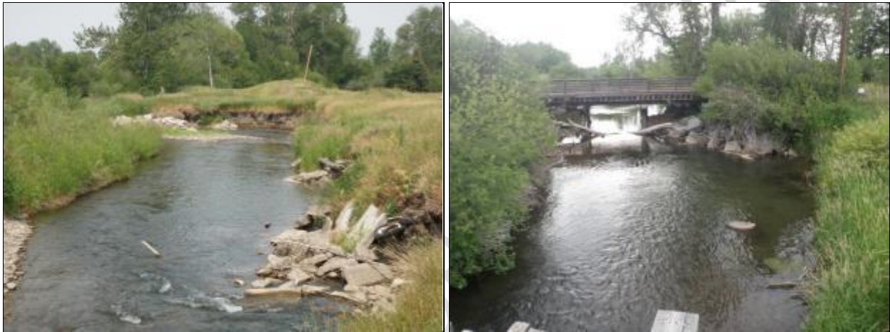
Figure 0-16. Existing bank armoring and bridge impacts on the East Gallatin River.
