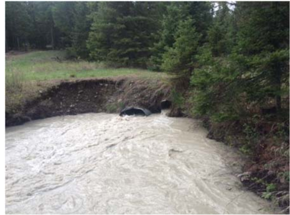
Figure 40. Undersized culvert during spring runoff.
