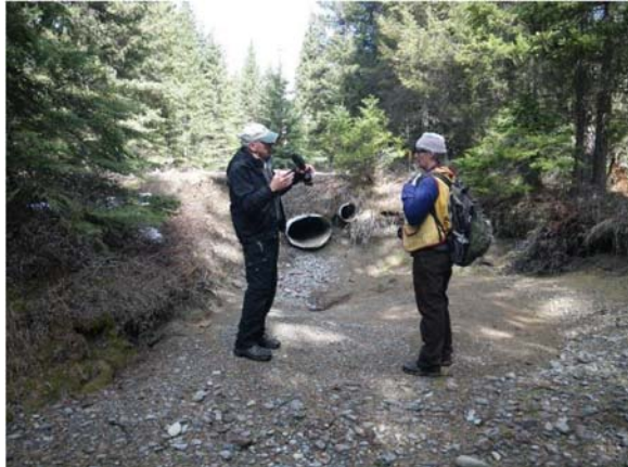
Figure 39. Undersized culvert.
