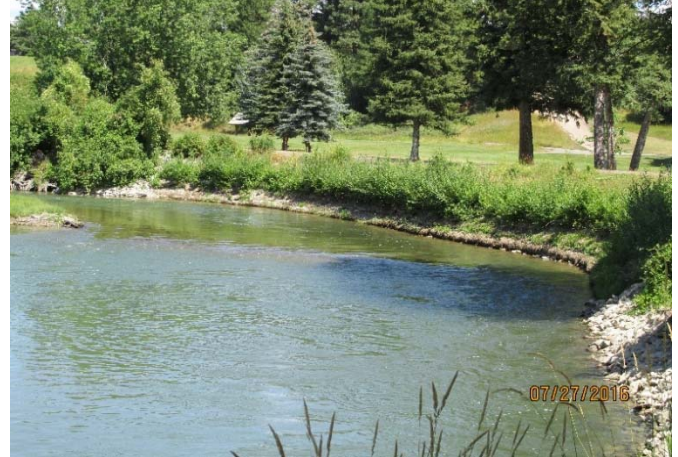
Figure 48. Same willow lift with willows growing out of the top layer and rip rap at the toe.
