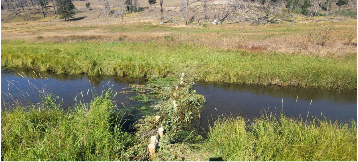
Figure 5: beaver dam analog. These structures simulate beaver dams; slow down and spread-out water which improves nutrient uptake and creates fish and wildlife habitat.
