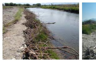
EXAMPLES OF WOODY DEBRIS MATRIX STREAMBANK TREATMENTS
