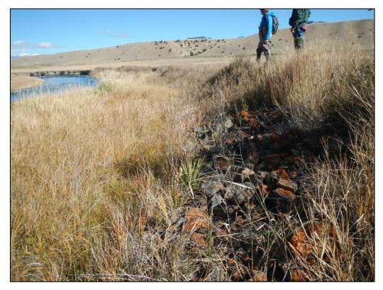
Figure 26. View downstream at RVHA showing old perched riprap.
