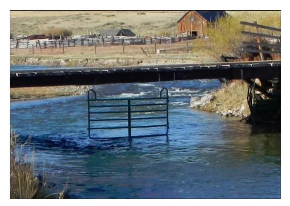
Figure 24. View upstream through bridge on south RVHA boundary showing an over-steepened area reinforced by rock riprap.
