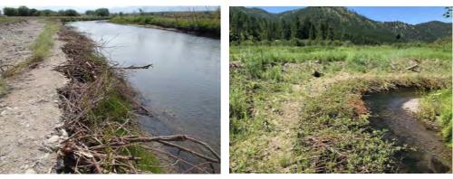
2. FOR TYPE 2 INSTALL BRUSH TOE FASCINE AND ANCHOR TO BACK OF EXCAVATION. FOR TYPE 3 CONSTRUCT STREAMBANK TOE WHERE NEEDED INSTALL WHOLE WILLOW CLUMPS IN THE STREAMBANK AT A DOWNWARD
