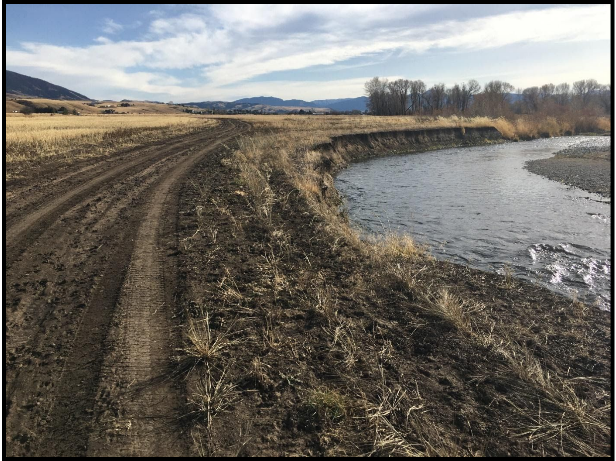
Photo 1. Looking upstream at Bank 2 (see Sheet 2), showing the agricultural encroachment on the river right bank, the existing unimproved road on the bank, and the vertical, unstable, poorly vegetated bank with an unnaturally high erosion rate. This is a candidate bank for bioengineered bank restoration and revegetation, and floodplain / riparian expansion.
