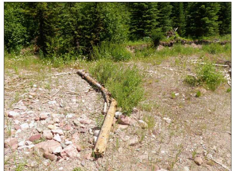
EXAMPLE OF A CONSTRUCTED VEGETATED BRUSH TRENCH
