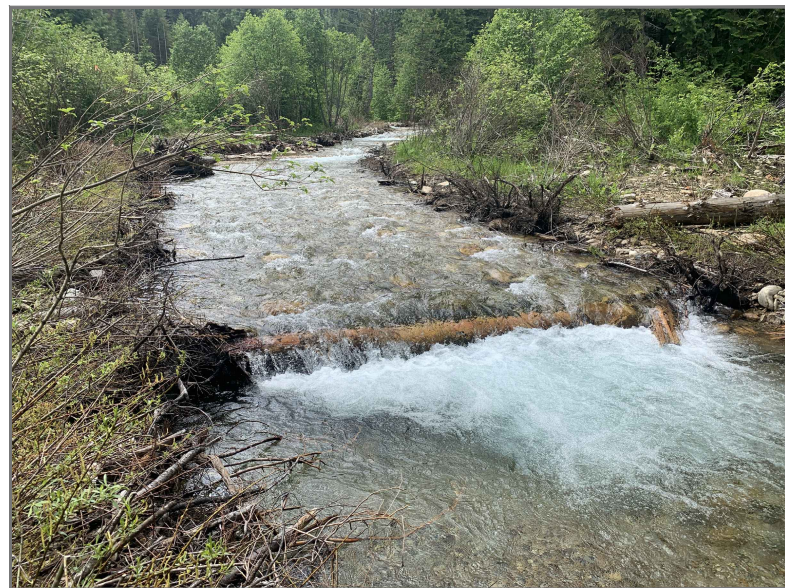
TYPICAL CONSTRUCTED STREAMBED THROUGH A RIFFLE FEATURE
