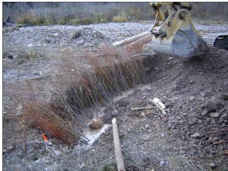
EXAMPLE OF A VEGETATED BRUSH TRENCH INSTALLATION
