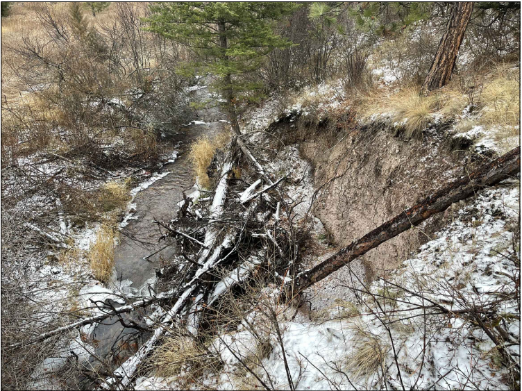
PHOTO OF EXISTING ROTATIONAL SLOPE FAILURE AT STATION 30+35
