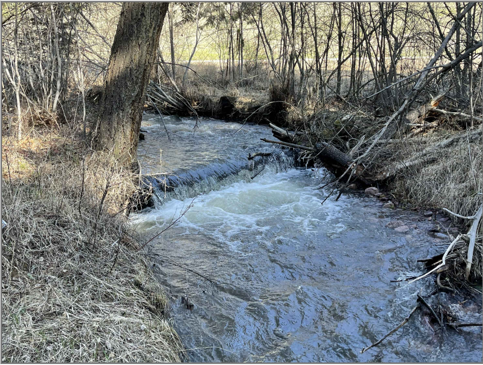
EXAMPLE OF A CONSTRUCTED LOG STEP POOL
