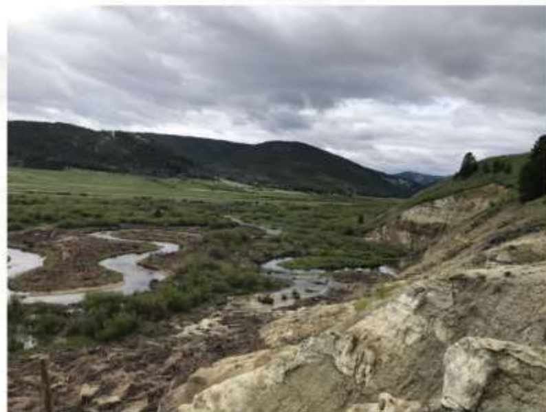
A photo of the completed project. Notice how the stream is moved away from the high, eroding hillslope, and wetlands remain. (Photo provided by the Big Hole Watershed Committee)
