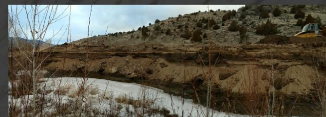
A rock structure installed to induce meandering.
