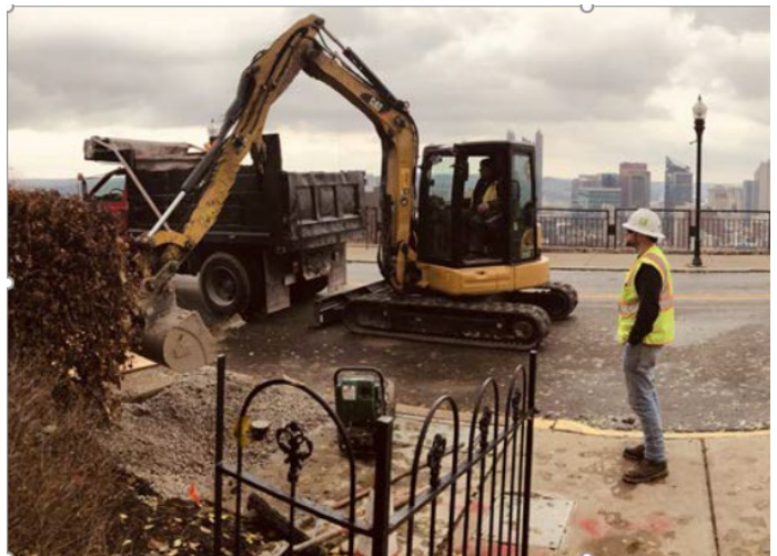
Example of a Mechanical Excavation
