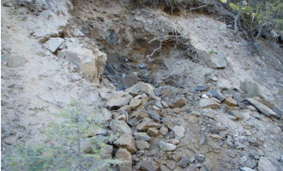
Photo 9: 09-MHRDTP-5 Looking West at the pit.
