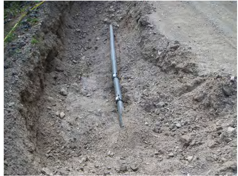
Photo 48: Mike Horse Creek Road repair pit & pipe repair (looking S).
