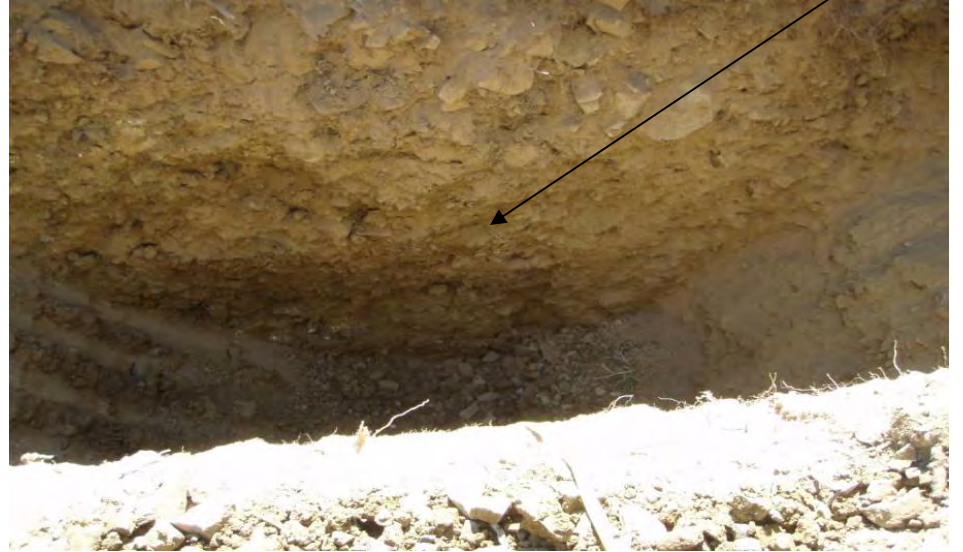
Photo 10: 09-SGTP-9 looking North. Highly weathered diorite in the test pit.
