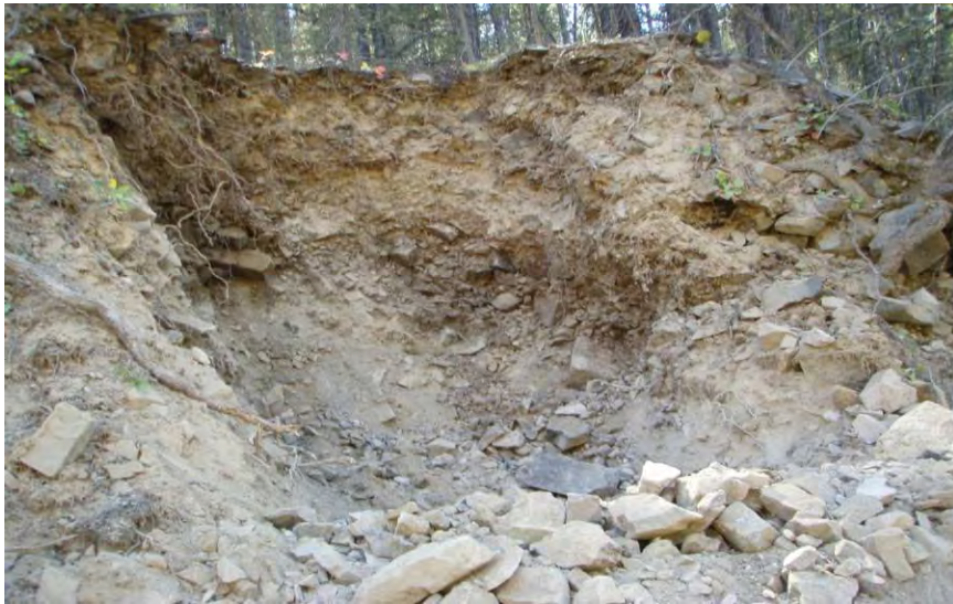
Photo 11: 09-MHRDTP-6 Looking North at the pit.
