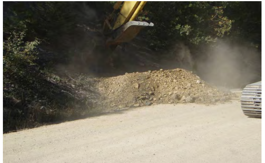
Photo 4: 09-MHRDTP-2 Looking North at pit and pile.
