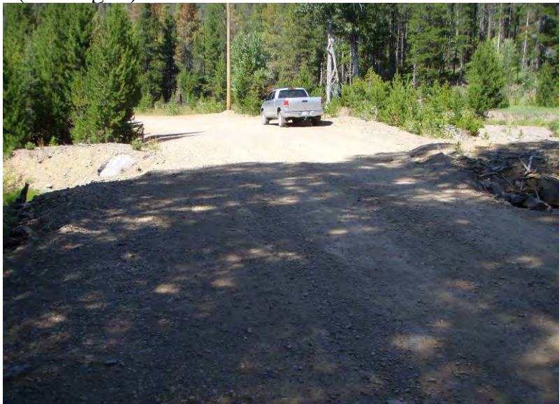
Photo 19: 24" CMP on Mike Horse Creek Road with 54" RCP (looking N).
