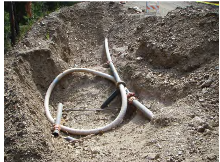
Photo 46: Same location as photo 45, pipe in the excavation (looking E).
