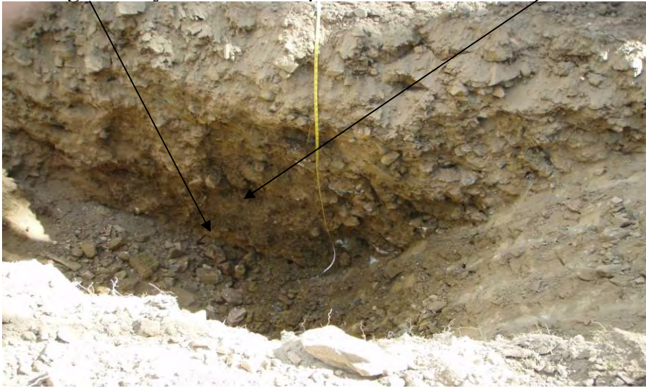
Photo 1: 09-SGTP-1 looking South. Highly weathered diorite and argillite layers in the test pit.
