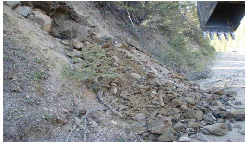
Photo 10: 09-MHRDTP-5 Looking North at pit and pile.
