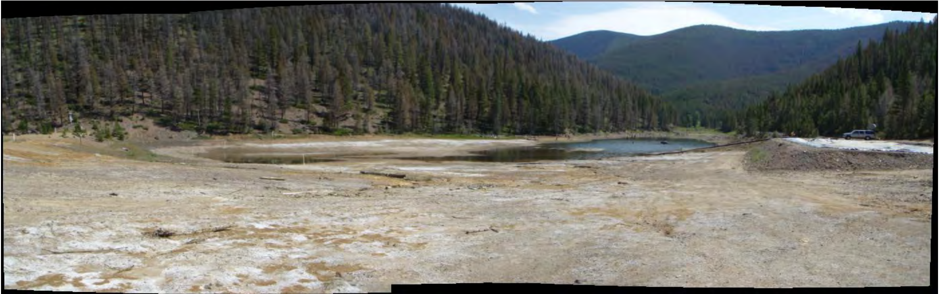
Photo 41: Panorama of Mike Horse Tailings Impoundment looking S from the dam.
