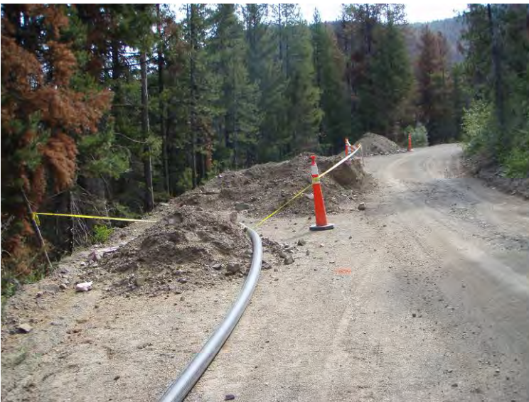
Photo 45: Mike Horse Creek Road pipeline & repair pit (looking E).
