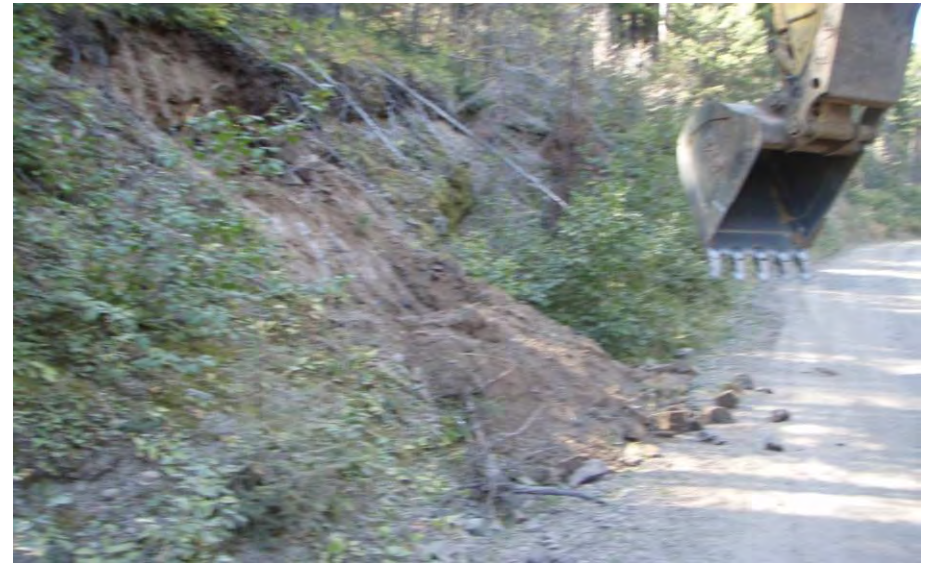
Photo 8: 09-MHRDTP-4 Looking North at pit and pile.
