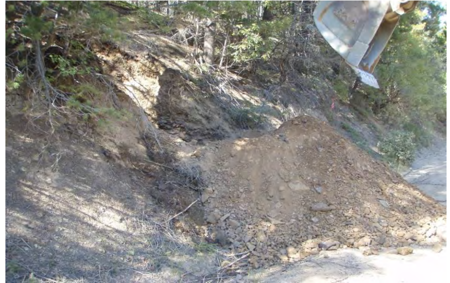
Photo 2: 09-MHRDTP-1 Looking North at pit and pile.
