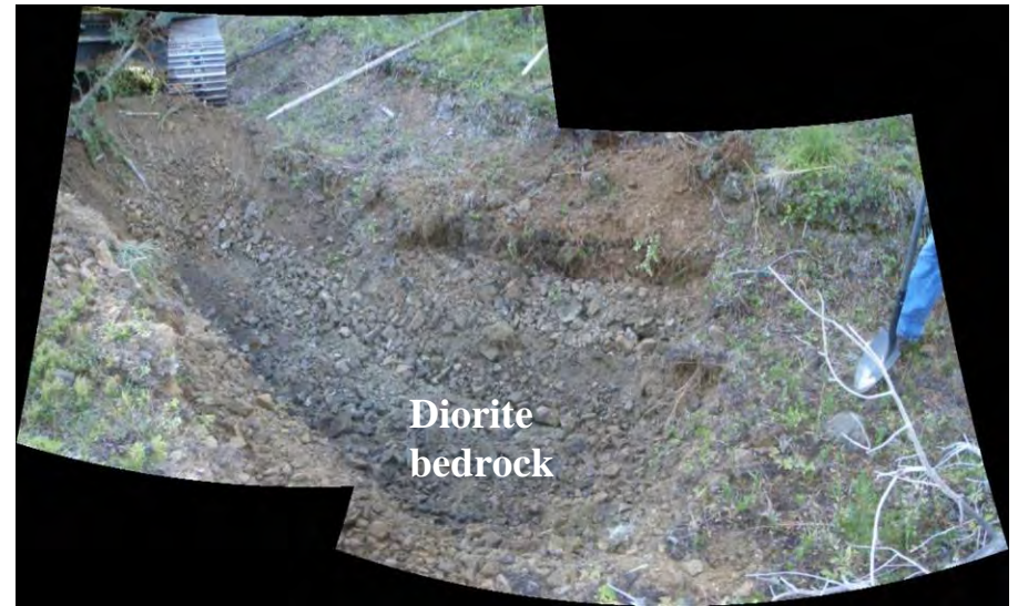
Photo 2: 09-PMTP-2 looking west into the pit.
