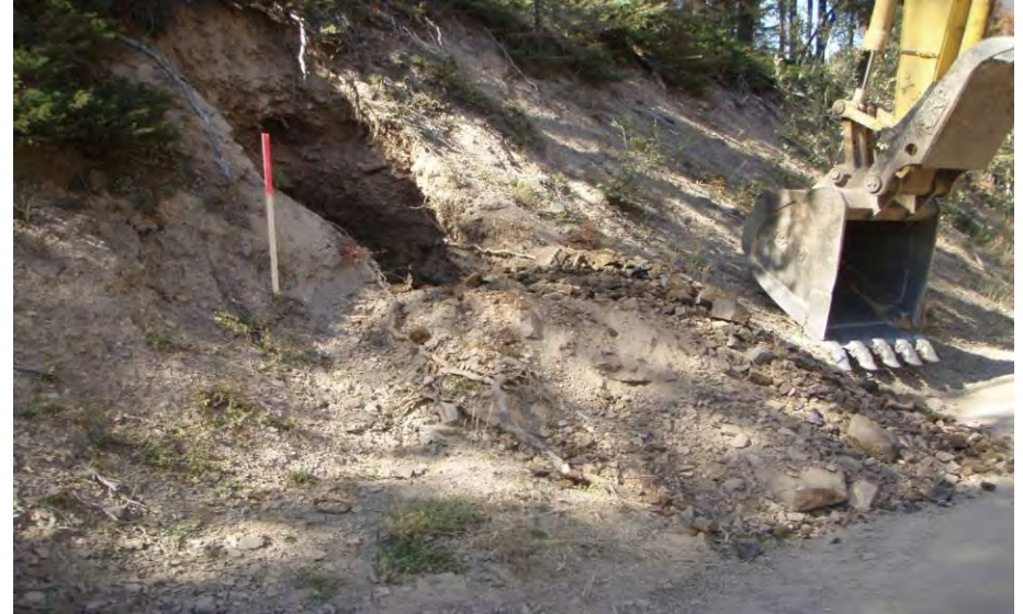
Photo 6: 09-MHRDTP-3 Looking West at pit and pile.
