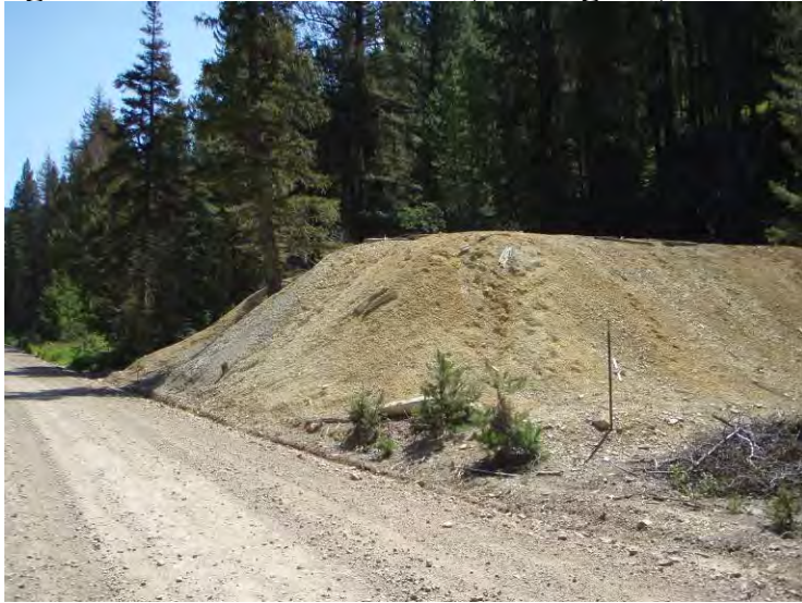
Photo 1: Waste/Tailings Pile below collapsed Mary P adit along Mike Horse Creek Road (looking SE).
