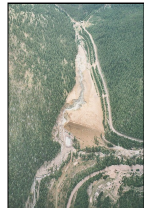
Dam breach in 1975
