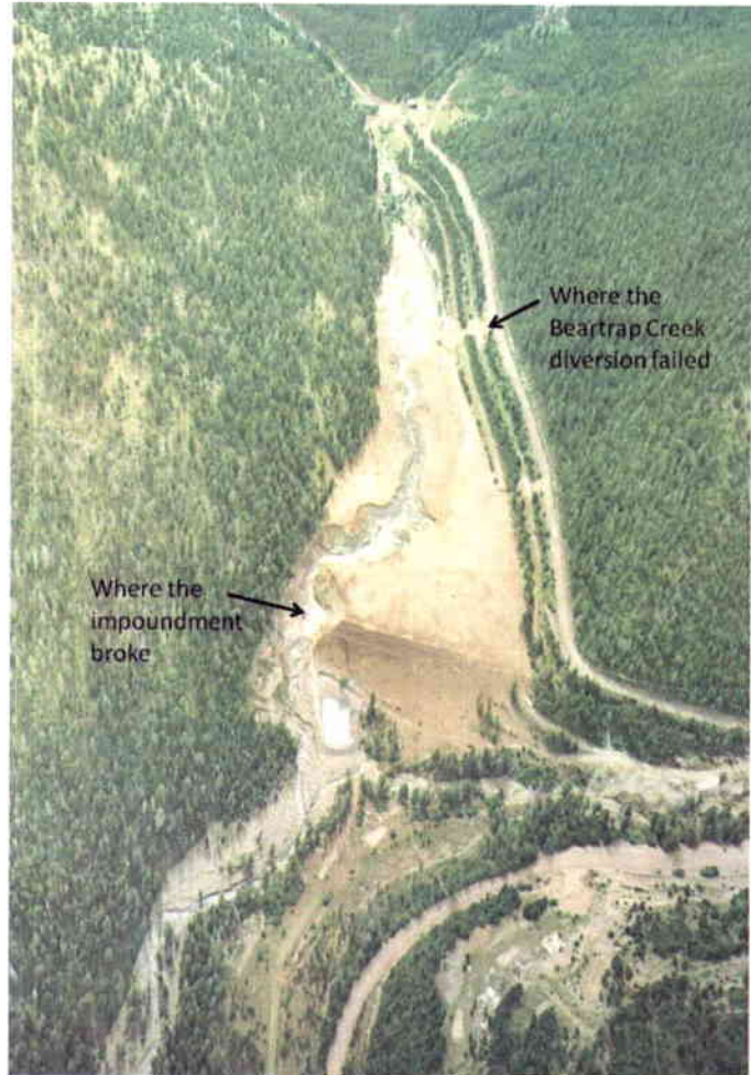
1975 dam breach - Beartrap Creek washing tailings into the Upper Blackfoot River
