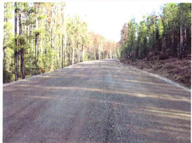
Newly constructed Meadow Creek Road
