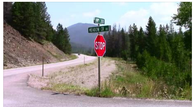
Trucks will be turning west from Meadow Creek Road onto Highway 279. Oncoming traffic has limited visibility.
