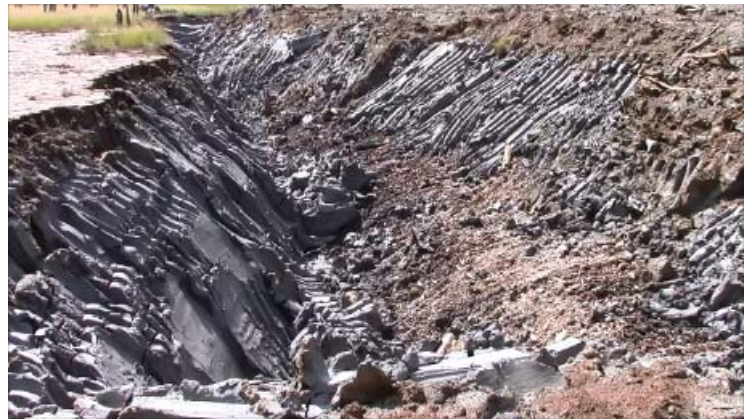
Excavation of mine waste from behind the Mike Horse impoundment.
