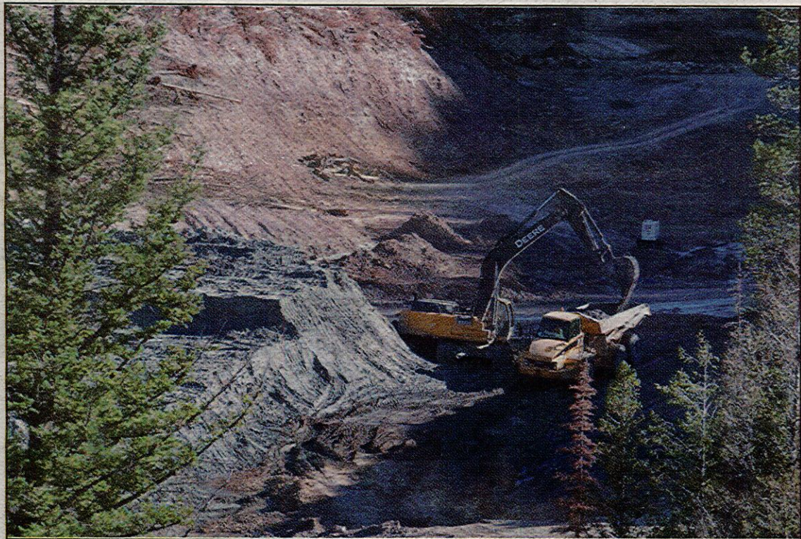
An excavator loads a dump truck with mine waste in the new gap in the remains of the Mike Horse dam.
