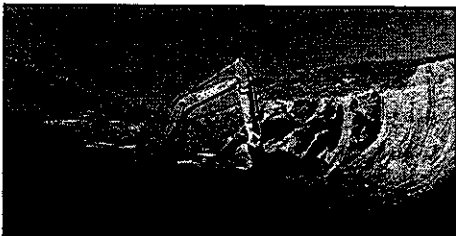
Looking north from the impoundment area as an excavator removes tailings where the dam once stood.
