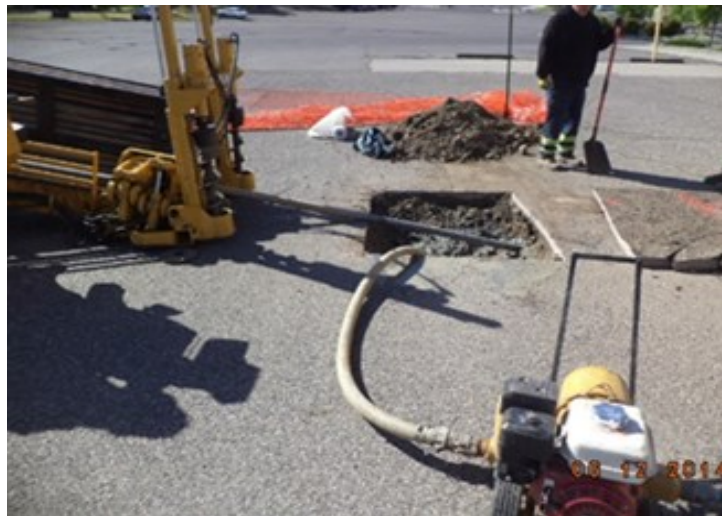
Installation of horizontal SVE wells.
