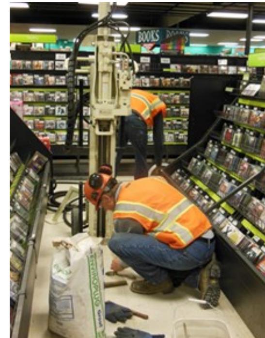
Soil vapor probe installation in the Hastings Shopping Center.
