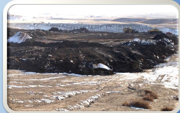
Waste material being spread at a TENORM landfill.
