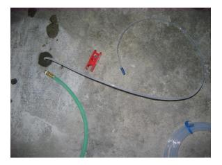
Cut the Teflon tubing, leaving approximately 3-4' of tubing above the top of the slab (enough for easy connection to the Summa canister). Place the end cap on the tubing. Allow the hydraulic cement to set for approximately 20 minutes or until hard to the touch.
