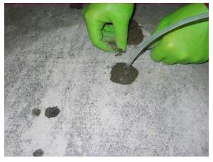
Cut the corner of the ziplock bag and squeeze cement into the final 1" of void space in the hole. Mound cement above the top of the slab and tightly around the tubing.
