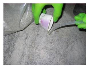
Put away the sand and begin adding the bentonite. At this point sand already should be above the bottom of the slab so there should only be 2-3" of void space in the hole, unless the slab is unusually thick. Add bentonite to approximately 1" below the top of the slab.
