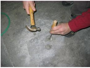
Put away all the equipment. Remove the concrete surface seal with a hammer and chisel. Using a finger or the end of a tool, compact the sand and bentonite in the sub-slab hole so as to avoid settling later.
