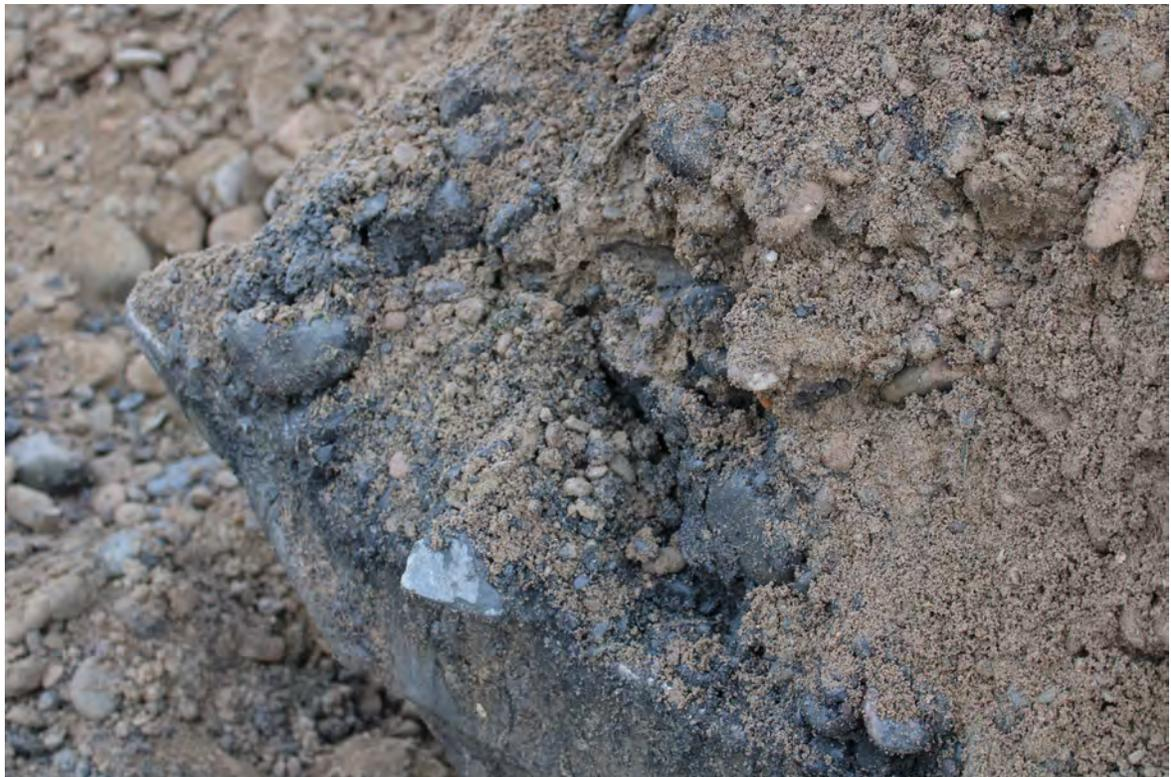
Photo 2. Pit run from the 2003 soil removal showing both the clean material above ~9 feet and the recontaminated material from 9 feet down. Slot trench from 28 Jan 2020.
