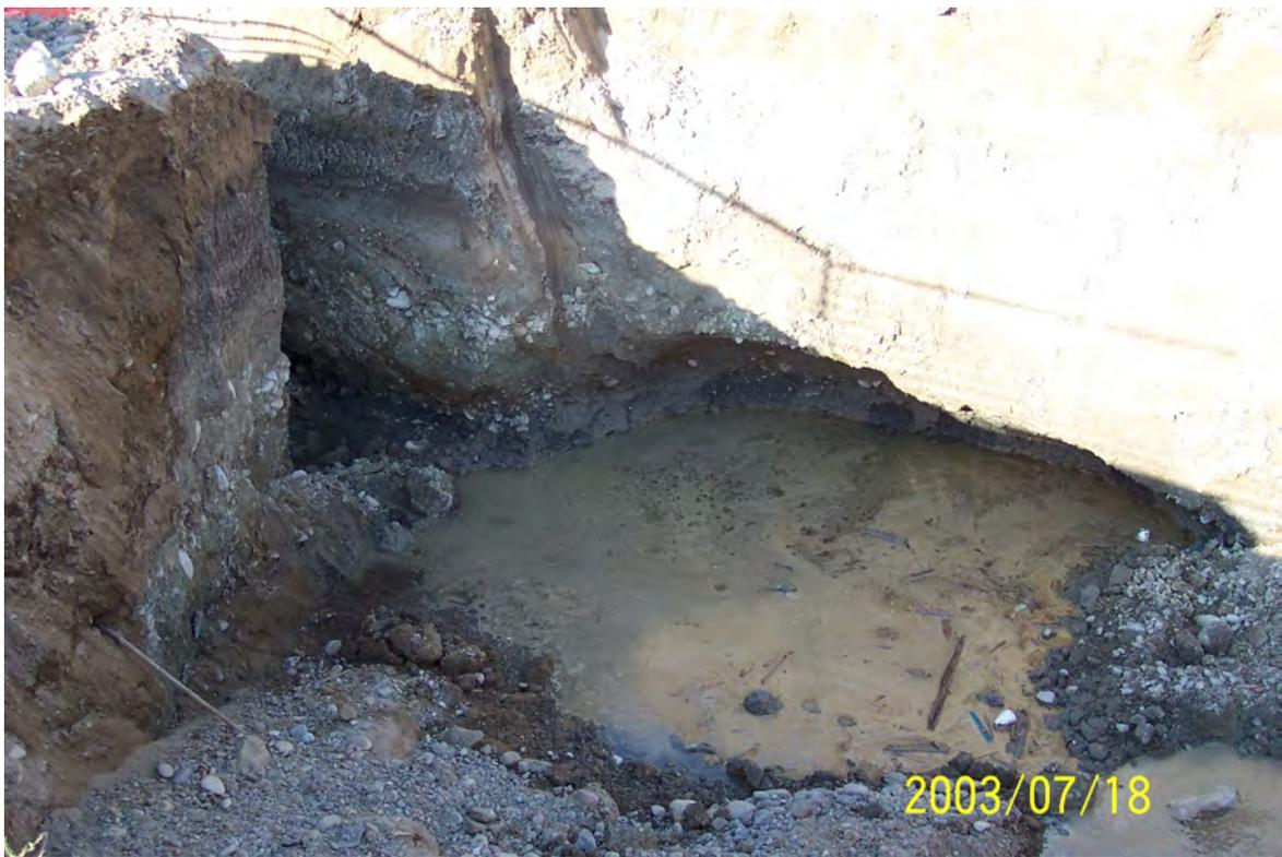
Photo 1. "Native soil " that was encountered during the 2003 soil removal. The zone of contaminated soil is easily determined by the color change and obvious odor of old fuel.
