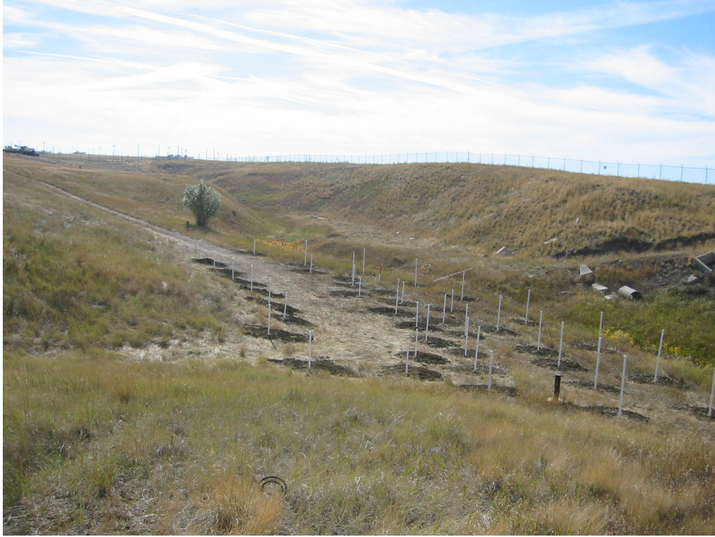
Installing a groundwater in-situ treatment system
